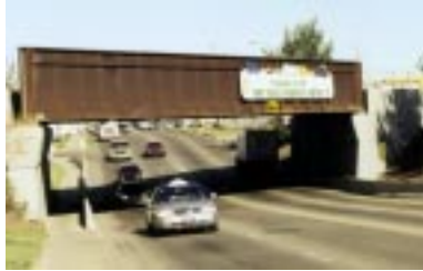
Fort Road view north under the CN train trestle.
