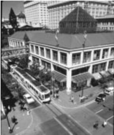
View of Portland Train Station Source: DPZ Associates
