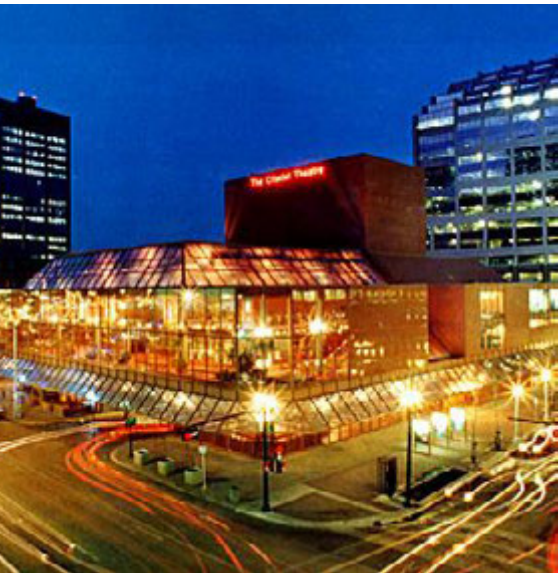
Photo courtesy Citadel Theatre
