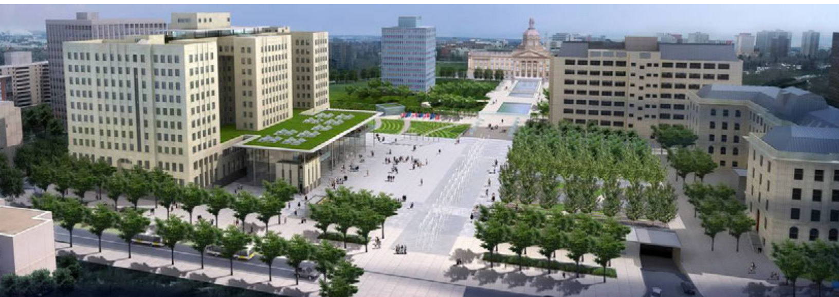
Image courtesy Carlyle + Associates
