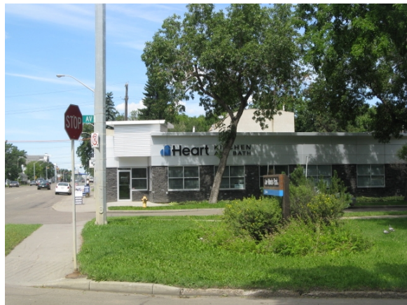
Joe Morris Park Frontage along 109 Street
