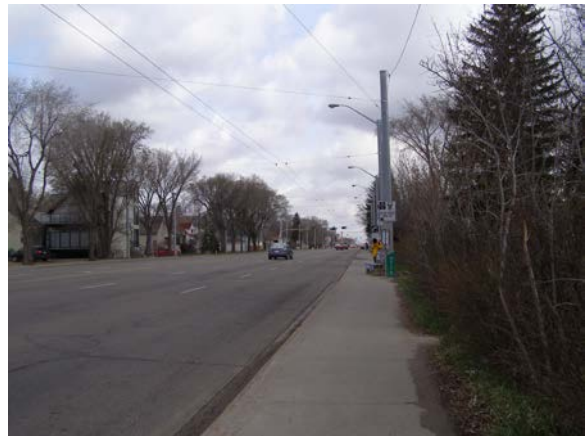
Narrow sidewalks and no boulevards, 109 Street
