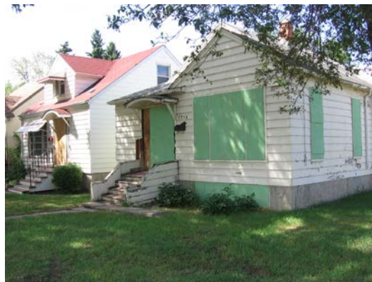
Vacant home along 109 Street
