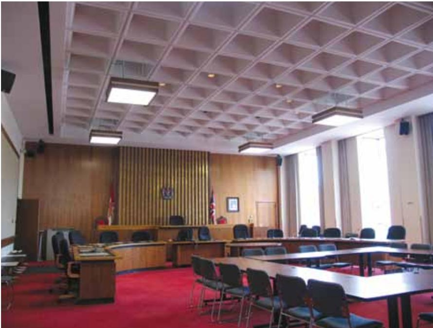
In modern buildings, reinforced concrete is often left exposed or simply painted in order to display a distinctive structural form, such as this waffle slab ceiling in the Victoria City Hall Annex. Inserting new wiring or services into such spaces can be challenging. Discreetly using conduit is recommended rather than installing false ceilings or walls that cover the historic structure.
