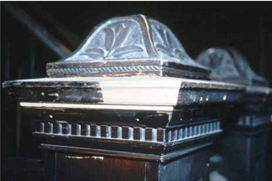
**Wood:** An example of “limited replacement in kind” describes an appropriate scope of work in the Preservation treatment. Only the damaged corner of a stair’s newel post at the Commissioner’s Residence in Dawson City, has been replaced (it will be stained to match). Only repairing deteriorated parts meant that most of the character-defining elements were retained.
