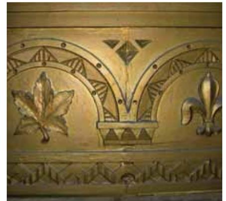
The repair of a deteriorated intricate plaster cornice should involve recognized conservation techniques, such as consolidation of the original materials in good condition. One goal should be to limit the amount of introduced material. Surface repairs may be filled with a compatible traditional plaster mix, but for larger elements, some form of adhesive or fastener may be required, and should be carefully selected.
