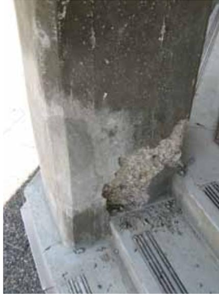
Deterioration of concrete is a significant conservation issue, particularly in the Canadian climate. Deterioration typically results from environmental factors, such as moisture, temperature and the presence of salts and carbon dioxide, which can corrode the steel reinforcements. Durability factors related to the original materials and workmanship, and improper maintenance, can also significantly affect concrete.
