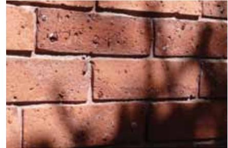
Sandblasting was once a popular method of removing paint from brick; however, it also removed the brick's outer hardened "crust" causing the brick to deteriorate.
