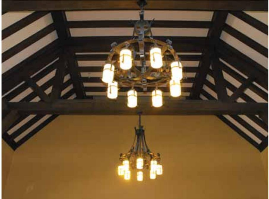
These large light fixtures in the main hall of the Jasper train station were rewired and adapted to accept compact fluorescent bulbs in order to meet sustainability and current health and safety concerns. Light fixtures of any scale can be similarly rehabilitated rather than being replaced.
