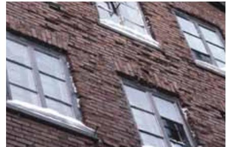
The harsh climate in many parts of Canada can seriously damage masonry elements. This wall has suffered irreversible damage from water penetrating the brick façade and freezing, causing the faces of many bricks to pop off. To avoid such damage, repair failed flashings, deteriorated mortar joints or other mechanical defects, but do not apply water-repellent coatings, which can trap moisture inside the masonry.
