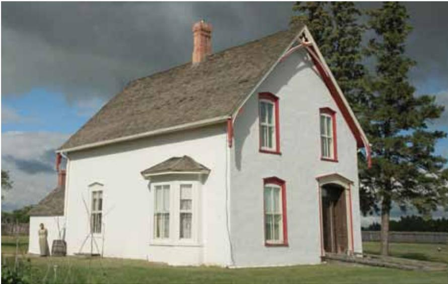
Before repairing or patching historic plaster or stucco, such as on the Commanding Officer's Residence at Fort Battleford NHSC in Saskatchewan, it is important to determine the composition of the material. Patches and repairs should be both visually and physically compatible with the existing historic material. Materials with different physical characteristics will likely not properly adhere to one another, necessitating repeated maintenance in the near future.
