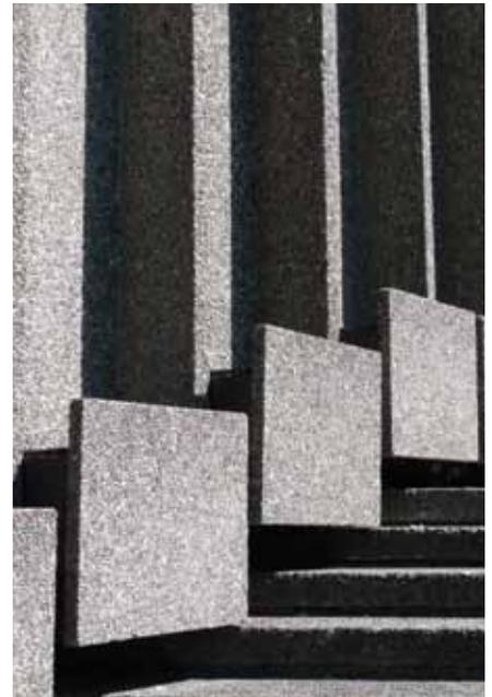
Special formwork or chemical or mechanical treatments can create a wide variety of concrete finishes, such as these pre-cast panels with exposed Laurentian granite aggregate at the National Arts Centre in Ottawa. Recreating these finishes when repairing or replacing-in-kind should be preceded by a mock up to ensure that the new work will be compatible with the historic place.
