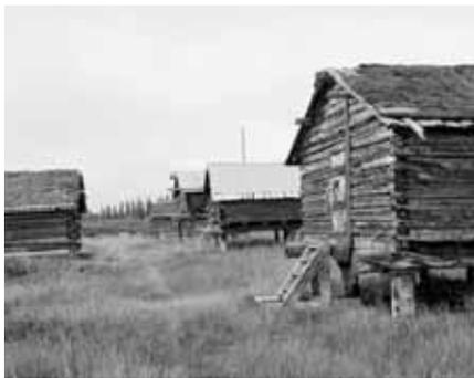
Sod was a simple, inexpensive and accessible roofing material used widely throughout the North and shown here at Knut Lang's place in the Northwest Territories. It is both waterproof and insulating and would last for decades before needing to be replaced. Frequently, when it began to fail, canvas was used as a temporary cover until a new sod layer could be applied.
