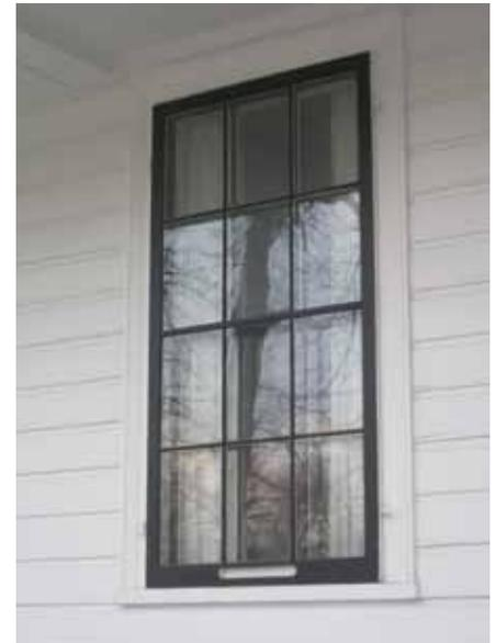
The type of glass and its division into multiple lights often defines the character of windows in historic buildings. The reflective quality of double-glazing from double sashes or storm windows is different than that of modern insulated glass. Inspections should be undertaken regularly to ensure that glazing putty is in good condition.
