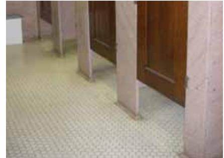
Mass-produced elements, such as ceramic tiles, are frequently used in buildings. Finding matching replacements for repair work can be almost impossible. If tile needs to be removed from one area, it is good conservation practice to save and stockpile it for later use elsewhere in the building. These tiles from the washrooms in Union Station in Toronto were removed from one set of washrooms in order to provide a stockpile of tiles to use in the repair of the remainder of the washrooms.
