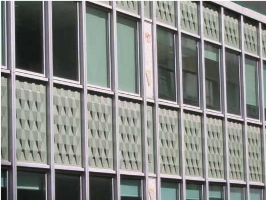
Plastic and fiberglass can be moulded into a variety of shapes to create decorative, colourful wall panels. These green moulded panels are unique and difficult to replicate if damaged. Removing intact panels from a less visible part of the building to replace broken panels in a more prominent area is one possible strategy.
