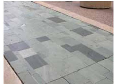
Deteriorated slate pavers should be replaced in kind from the same source of the original material. If the original quarry is closed, a suitable match should be located and attention given to the stone's composition, strength and colour.
