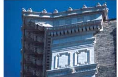
One of the primary causes of deterioration of glazed architectural terra cotta, like that shown on the Confederation Life Building in Winnipeg is water. Water-related damage to the glazed units, mortar, metal anchors or masonry backfill can be repaired only after eliminating the sources of that water. In order to ensure that the actual root problem is being solved, investigation work would need to be completed prior to any repairs in order to identify that source.
