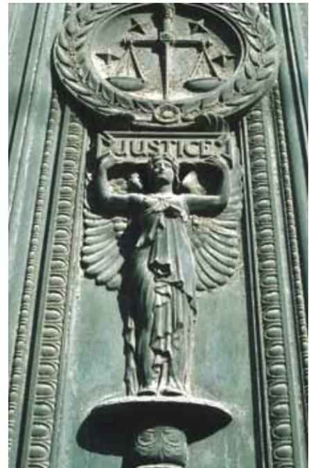
The first step in preserving architectural metals is to identify the type of metal. Before cleaning, determine that the method is appropriate for the particular metal: removing the patina from these bronze doors would not be appropriate if the patina is a character-defining finish of the metal, or if it provides a protective coating. Testing is recommended to ensure that the gentlest cleaning method possible is used.
