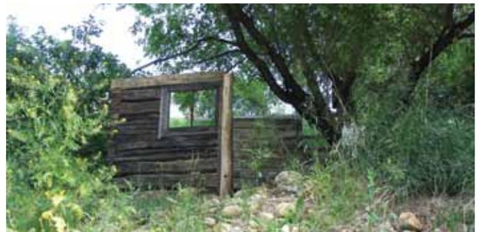
The character-defining elements of Doukhobor Dugout House NHSC in Saskatchewan, such as the window frames, had suffered visible deterioration from exposure to the elements. A long-term repair solution was necessary to prevent further decay and to preserve the site's heritage value.
