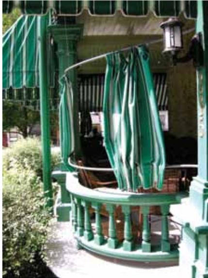
Fabric awnings are subject to damaging environmental effects including sunlight, wind and water, which eventually may cause the loss of the historic awning fabric. Repairing the original frame or mechanism and installing new awning fabric are recommended and will also help provide shade. Awning manufacturers may be able to match or provide similar fabrics compatible with the character of the place, as was done at Laurier House in Ottawa.
