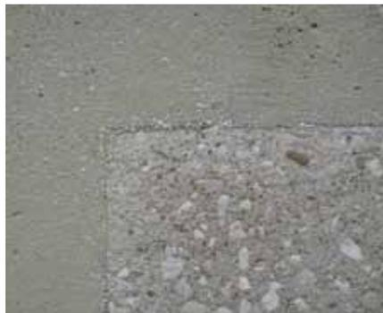
Important properties to match when patching concrete can include the modulus of elasticity, cement to aggregate ratio, aggregate gradation, compressive and shear strength, and coefficient of thermal expansion. In this case the coarse aggregate in the repair patch does not match that of the original concrete.
