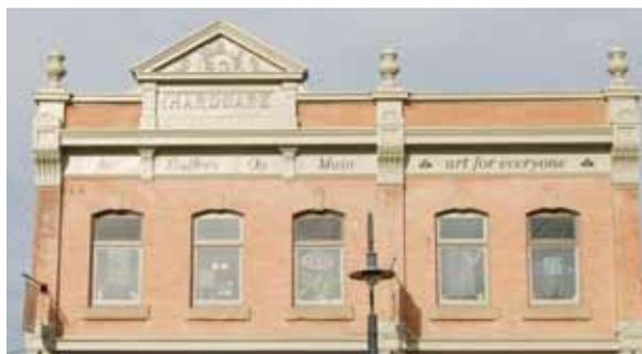
The two remaining decorative sheet metal urns at the top of the façade of the M & J Hardware Building in Lacombe, AB were determined to be beyond repair due to weathering over time. A third sheet metal urn (centre) was missing. The existing deteriorated elements and photographic documentation were used to replicate these elements. The M & J Hardware Building is an example where missing features from the restoration period have been re-instated based on physical and documentary evidence.
