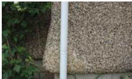
Certain stucco treatments, such as pebble-dash stucco, are difficult to replicate. Applying glass or rocky aggregate to the wet stucco is an art that is all but lost. Pebbles imported from Scotland for the Dr. Woods House in Leduc, AB are virtually impossible to replicate. The repairs resulted in a sound exterior envelope, but are clearly distinguishable from the original.
