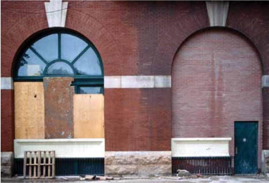
Masonry should be cleaned only when necessary to halt deterioration or remove heavy soiling. If surface cleaning is appropriate, test to select the gentlest cleaning method possible, and observe the result over time to determine the immediate and the long-term effects. Test cleaning the left portion of this brick and stone wall (using low pressure water and detergents, when there was no chance of freezing) created an acceptably clean wall.
