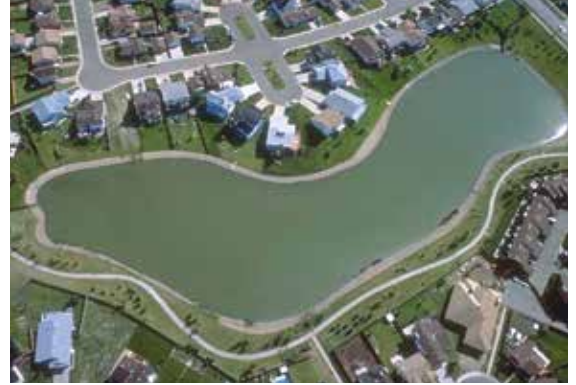
Stormwater Management Lake
