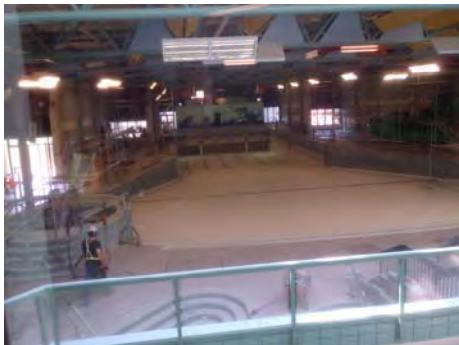
Mill Woods Recreation Centre – Pool Area Undergoing maintenance in Fall 2012
