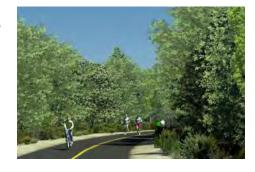
Enhanced Walking Trails – walking trails will be formalized and improved on some of the existing paths using compacted granular placed at 3.0 m wide for the main trails and at current widths for other informal trails, through forested
