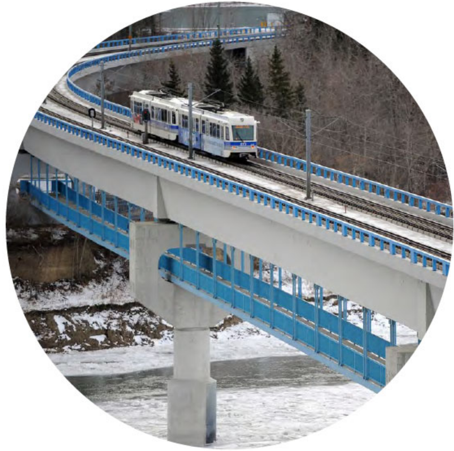
Edmonton Light Rail Transit (Dudley Menzies Bridge) 1978
