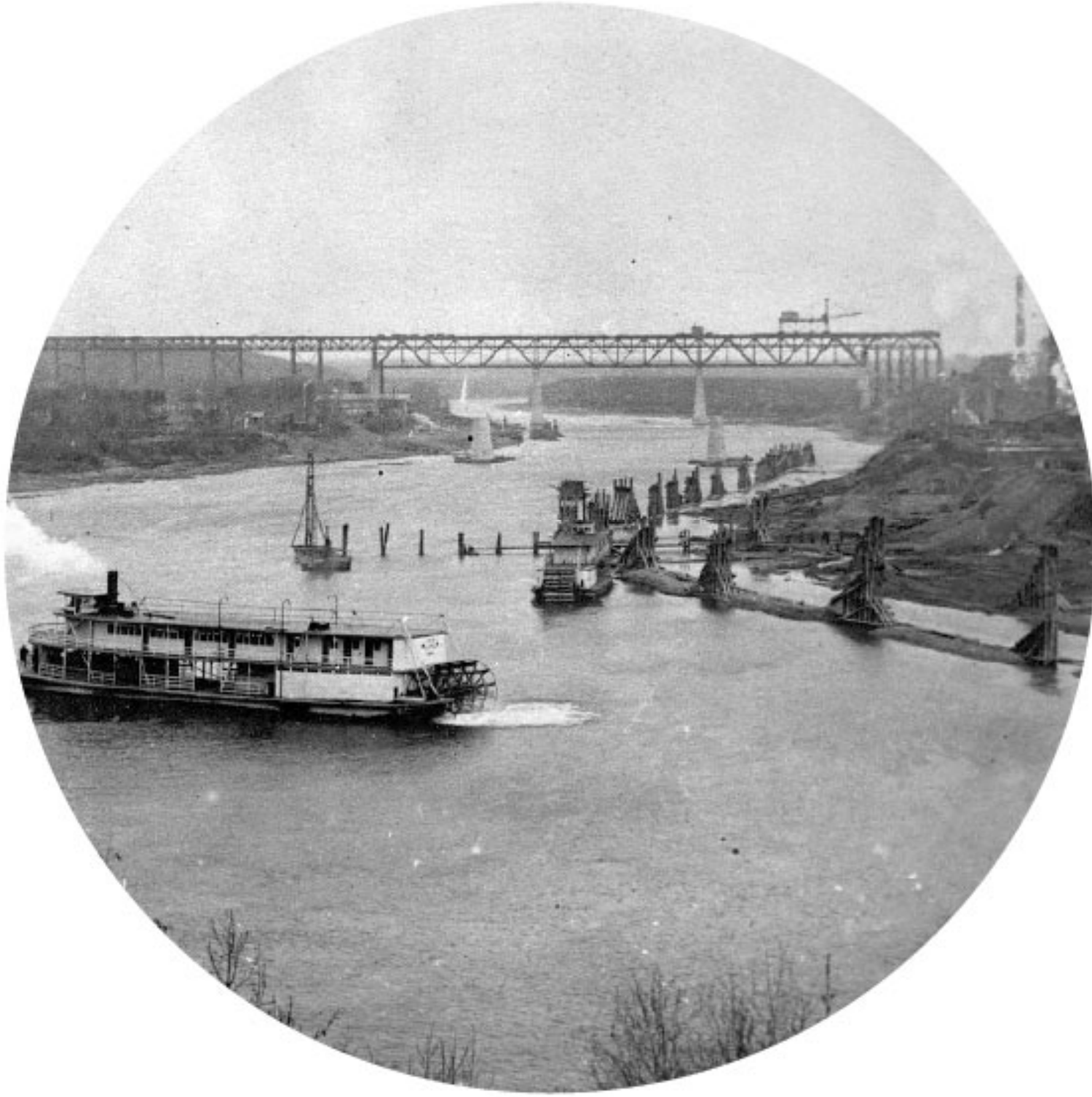
High Level Bridge under Construction 1912
