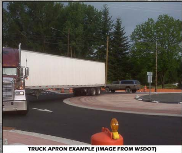
TRUCK APRON EXAMPLE (IMAGE FROM WSDOT)
