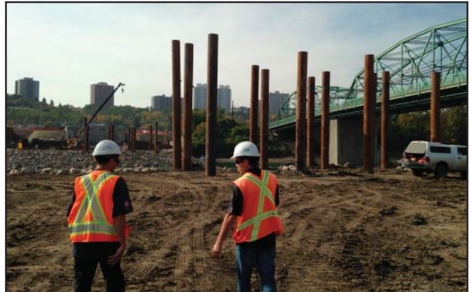
Pilings installed on north river berm.
