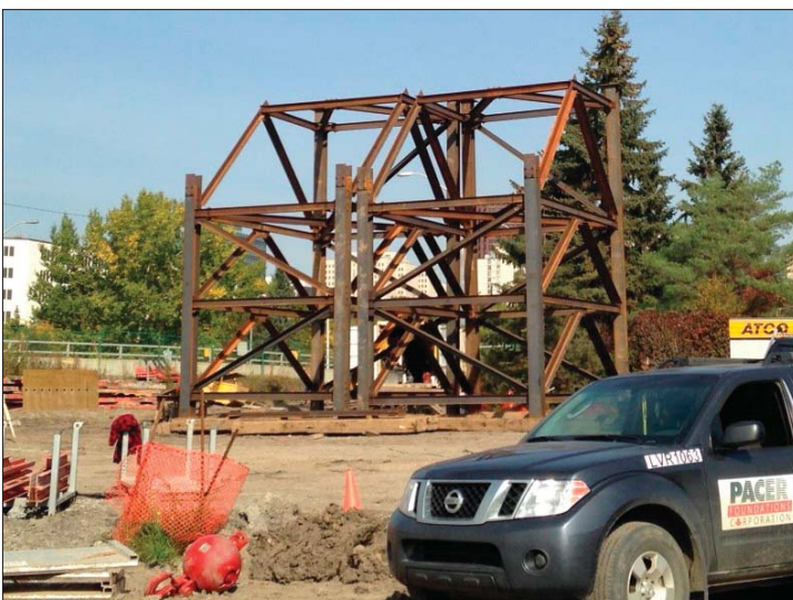
Tower assembly on the north side.
