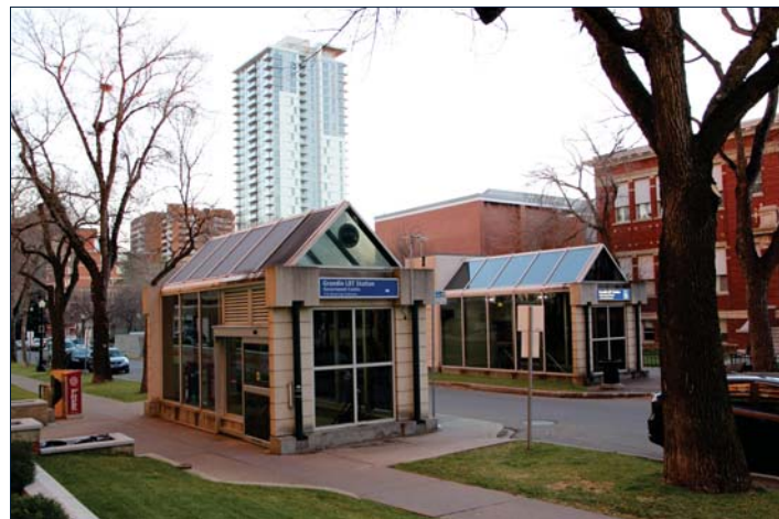
Pedestrian entrance at Grandin station
