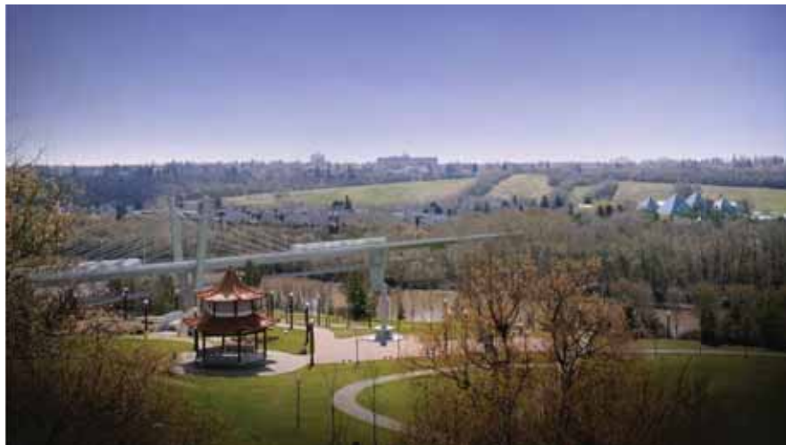
Extradosed bridge looking Southeast
