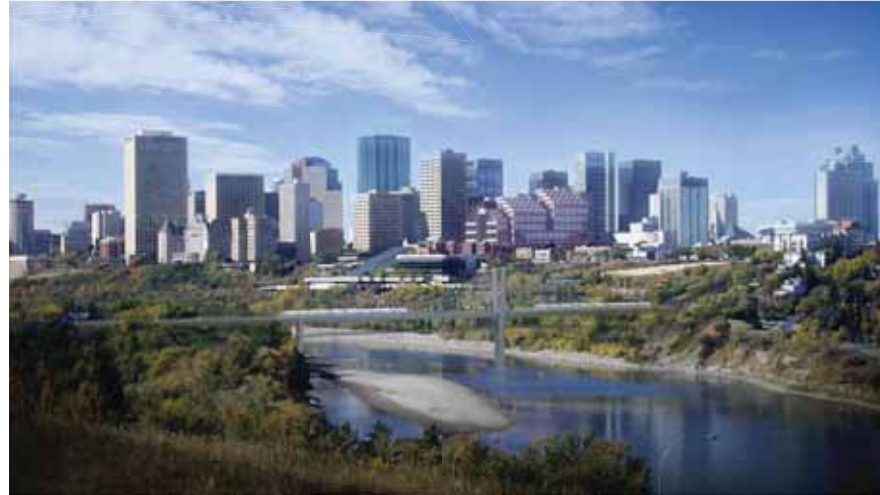
Extradosed bridge looking Northwest
