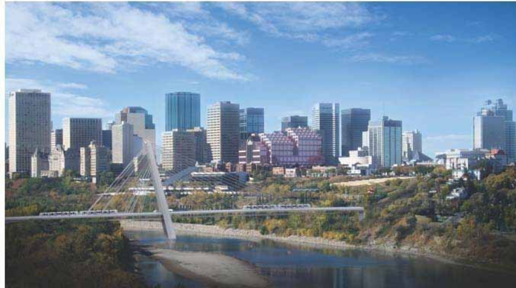
Option 1 - Cable stayed bridge looking Northwest
