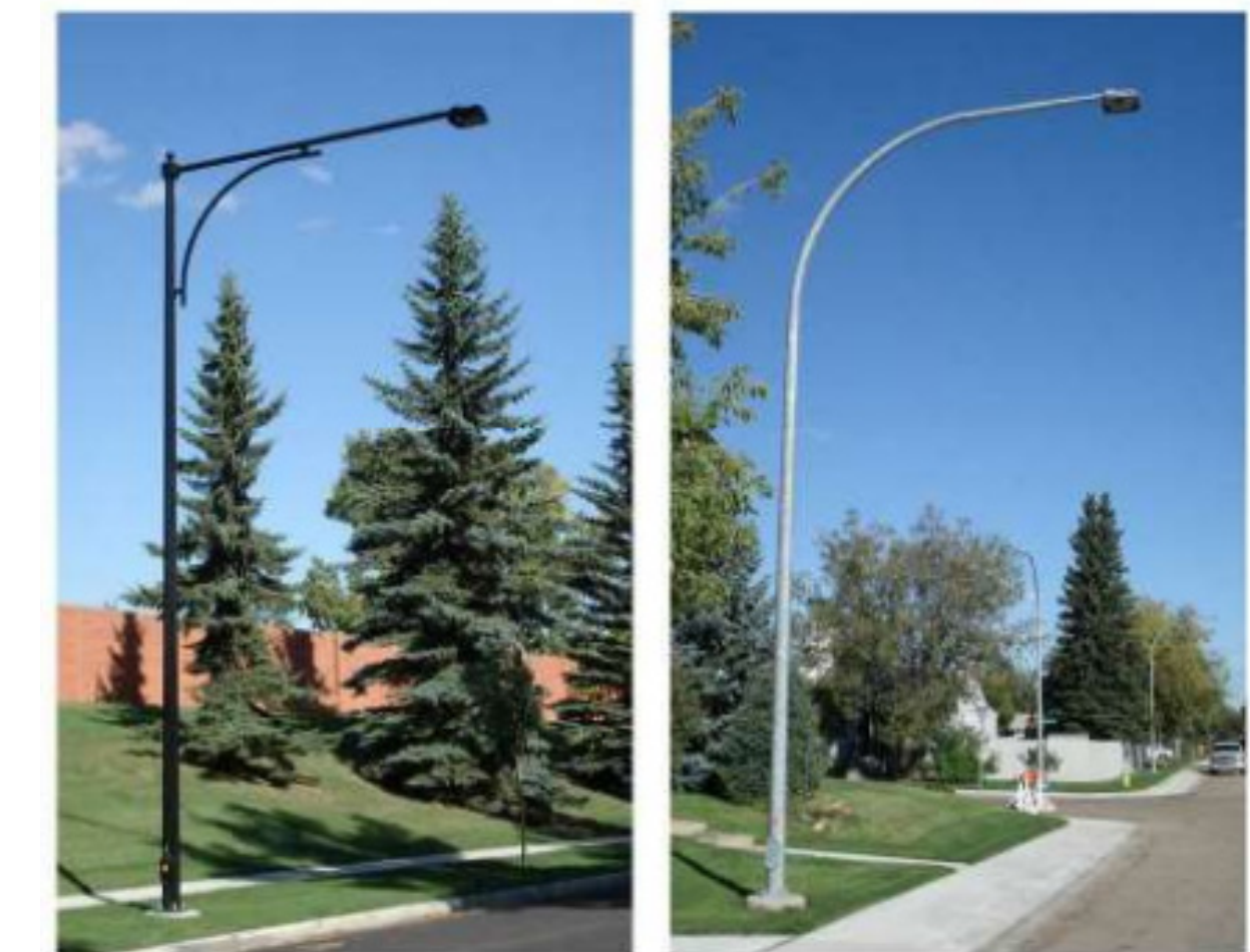
Decorative streetlight Standard streetlight
