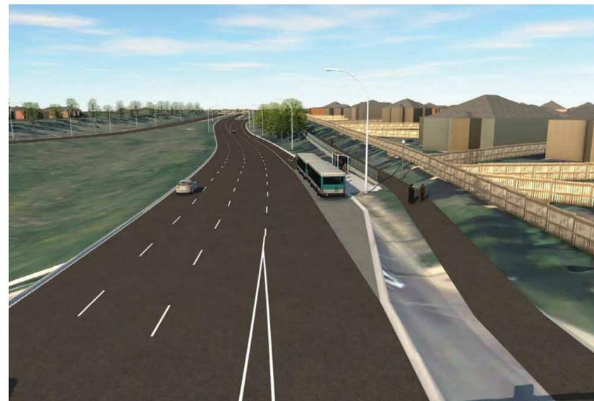
Concept of the separated bus lane at a bus stop.
