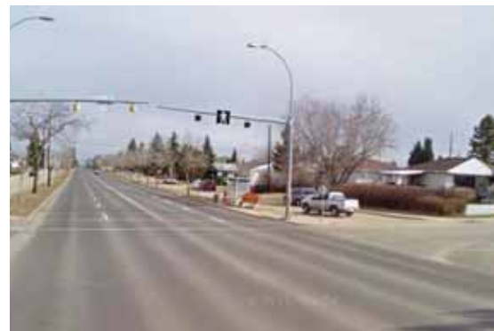
View A - Existing Condition
