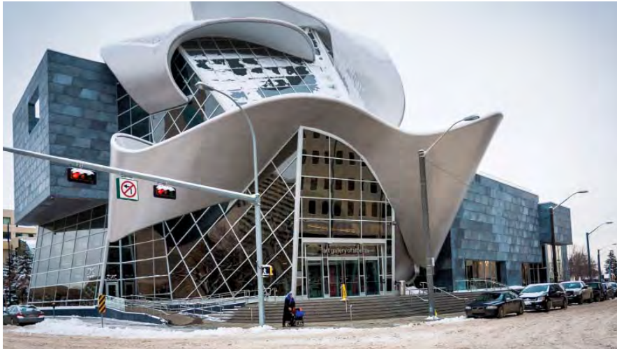
Variable roof shapes deflect falling snow and ice away from entrances, walkways and stairs, like at the Art Gallery of Alberta in Edmonton, AB ▲
