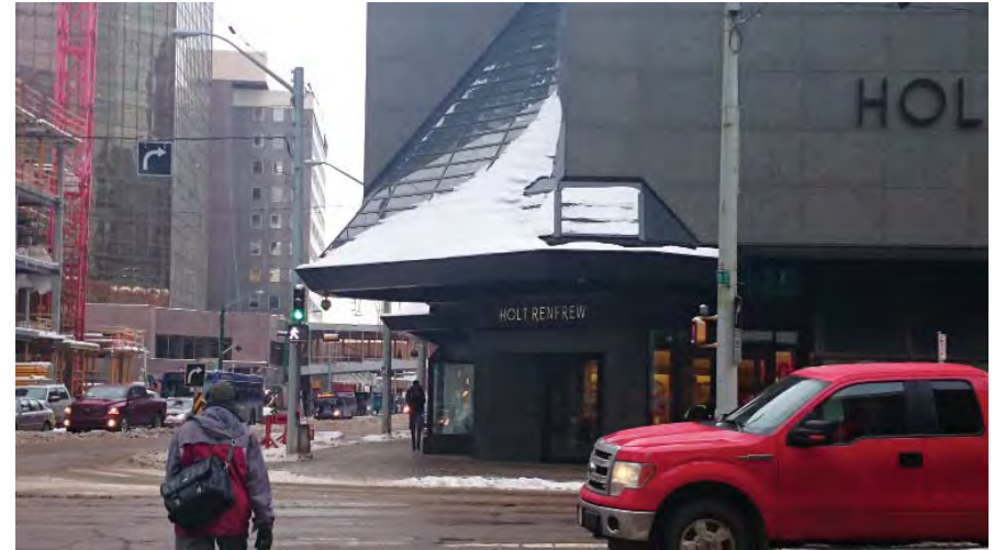
▲ Snow guards hold snow on a wind-drifted cornice at a retail entrance
