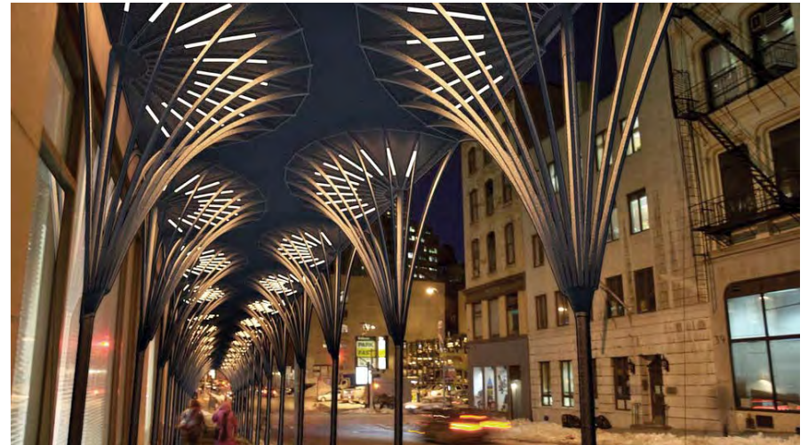
▲ Urban Umbrella, designed Young-Hwan Choi, Sarrah Khan and Andres Cortes, is artistic, yet functional, construction hoarding made out of recycled steel, translucent plastic panels and LED lighting in New York City, USA
