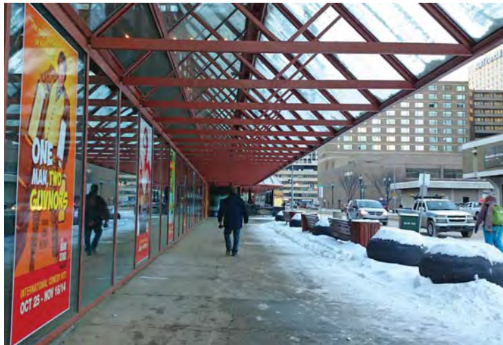
Durable, transparent materials allow for natural lighting. Canopy installations may require winter maintenance during the snowy season ▲
