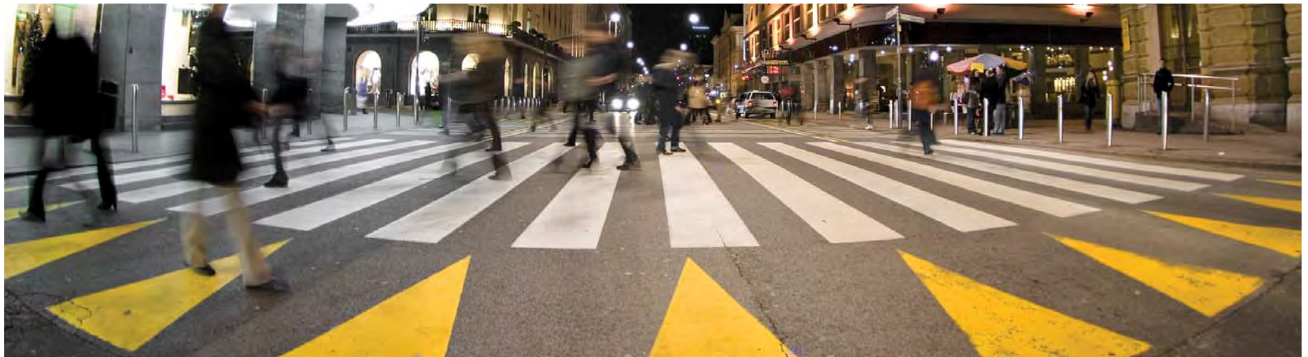
Reflective zebra-striped street crossing, with appropriate coloured road surface markings, clearly indicates a speed table and pedestrian crossing area ▲
