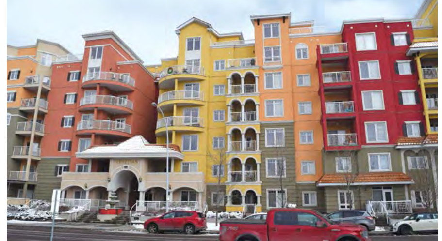
▲ The appearance of a city can be changed significantly with colourful buildings, such as The Venetian in Edmonton, AB
