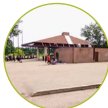
100 pavilion minor improvements
