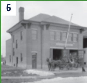
6 Former Firehall # 8 10986-126th St. Served the surrounding area for over 50 years (Glenbow Archives - ND-3-414)
