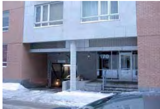
Minimal impact parking garage entrances
