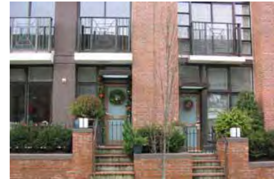
Front doors with street address and main floors no more than 1.0m higher than the public sidewalk
