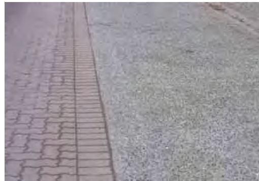
Crosswalk paving treatment - Example
