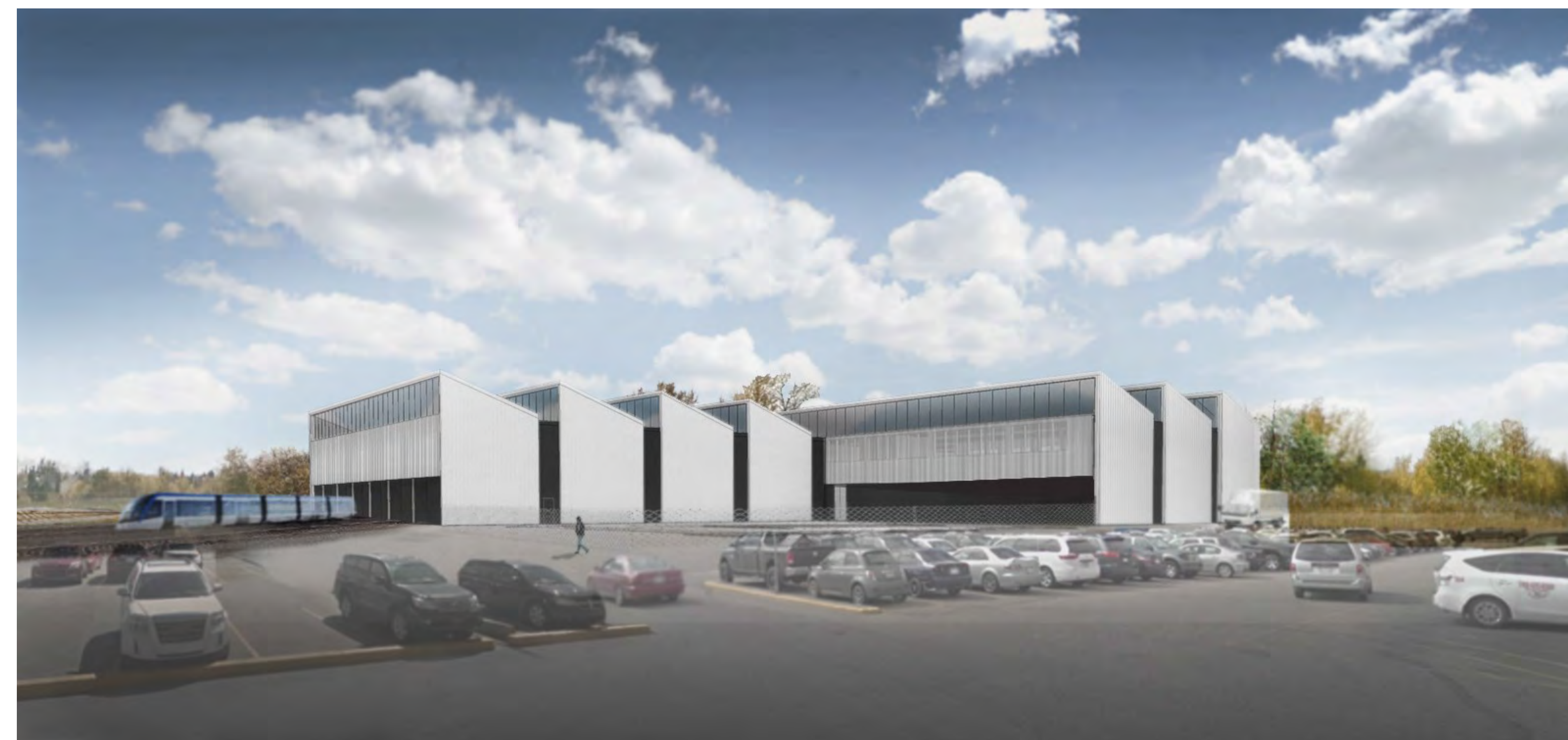
LRV storage facility viewed from the northwest
