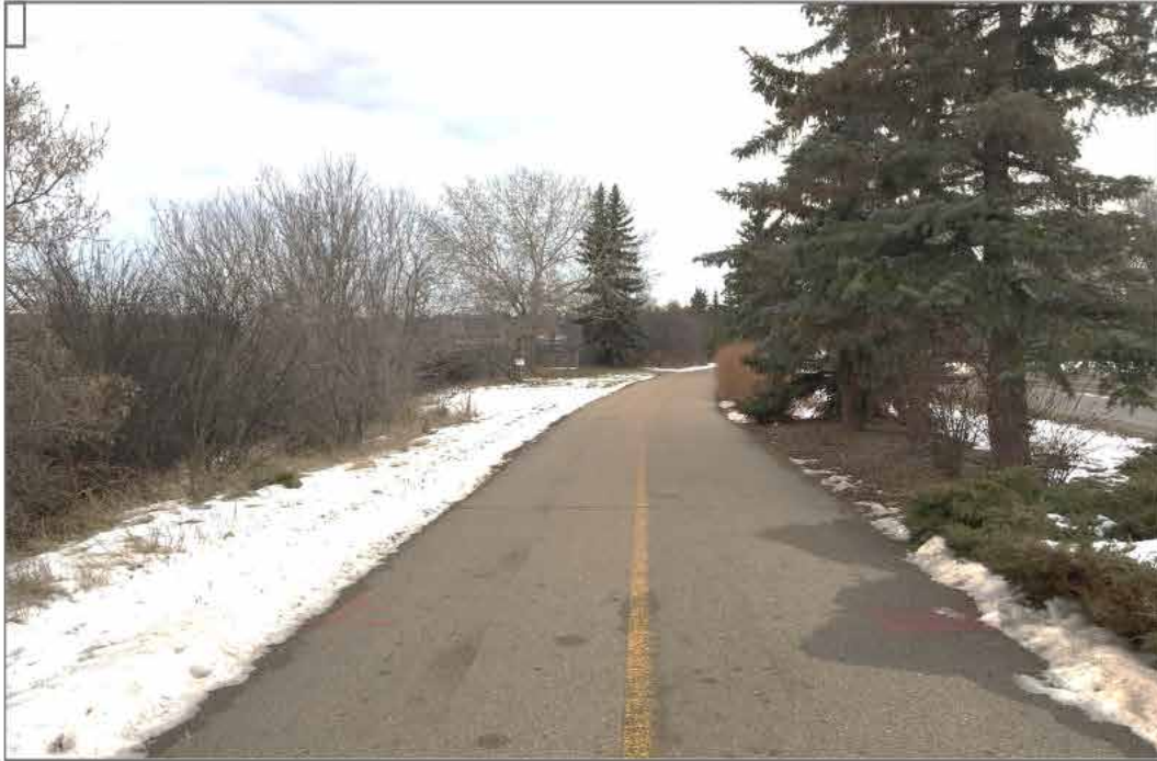
Photo 3: Eroded Channel on River Bank Slope
