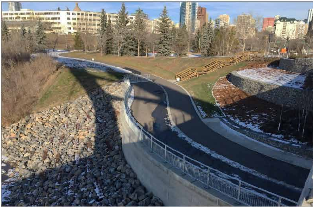
Photo 17: Existing Retaining Wall and Trail near Waltherdale Bridge (Looking West)
