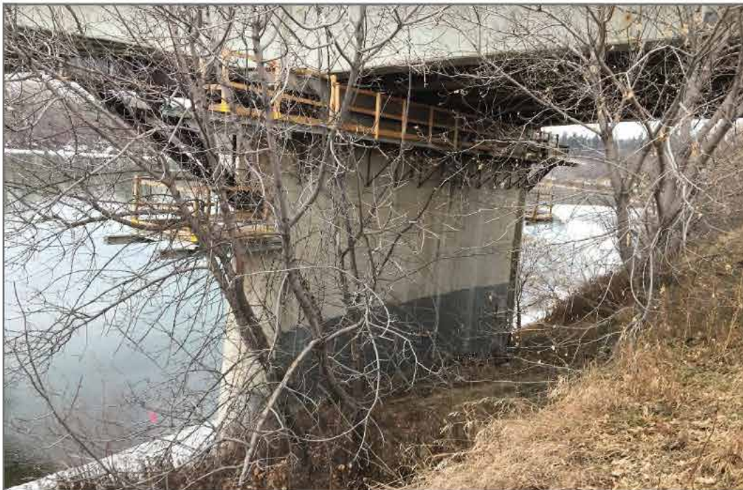
Photo 4: Groat Road Bridge Pier at Slope Toe
