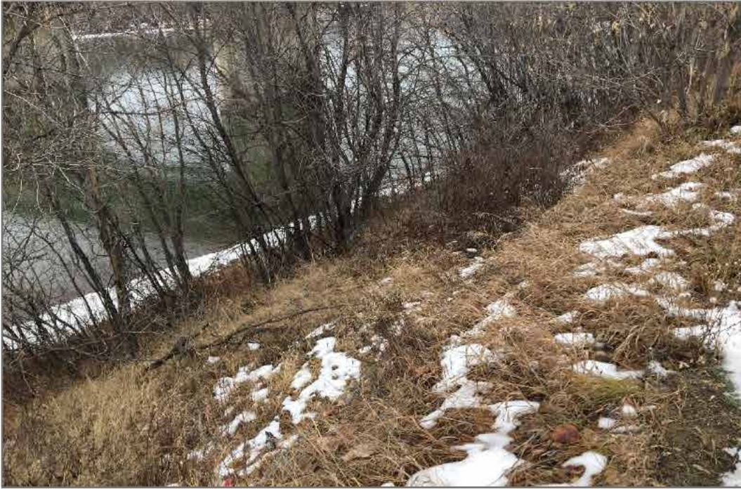
Photo 5: Existing Buried Gabion Wall at Top of River Bank Slope
