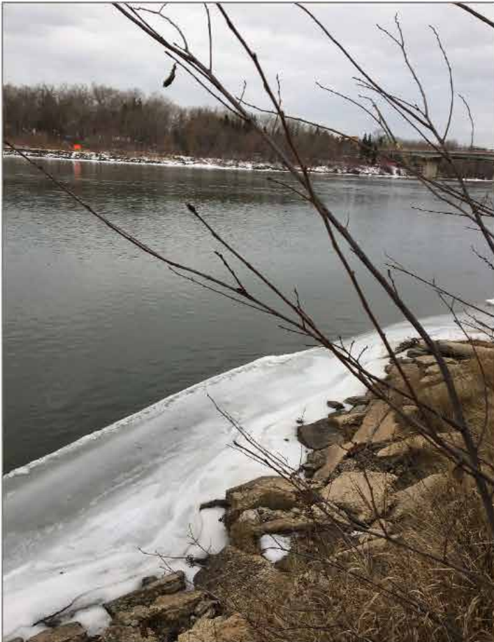
Photo 13: Large Concrete Blocks close to River Level
