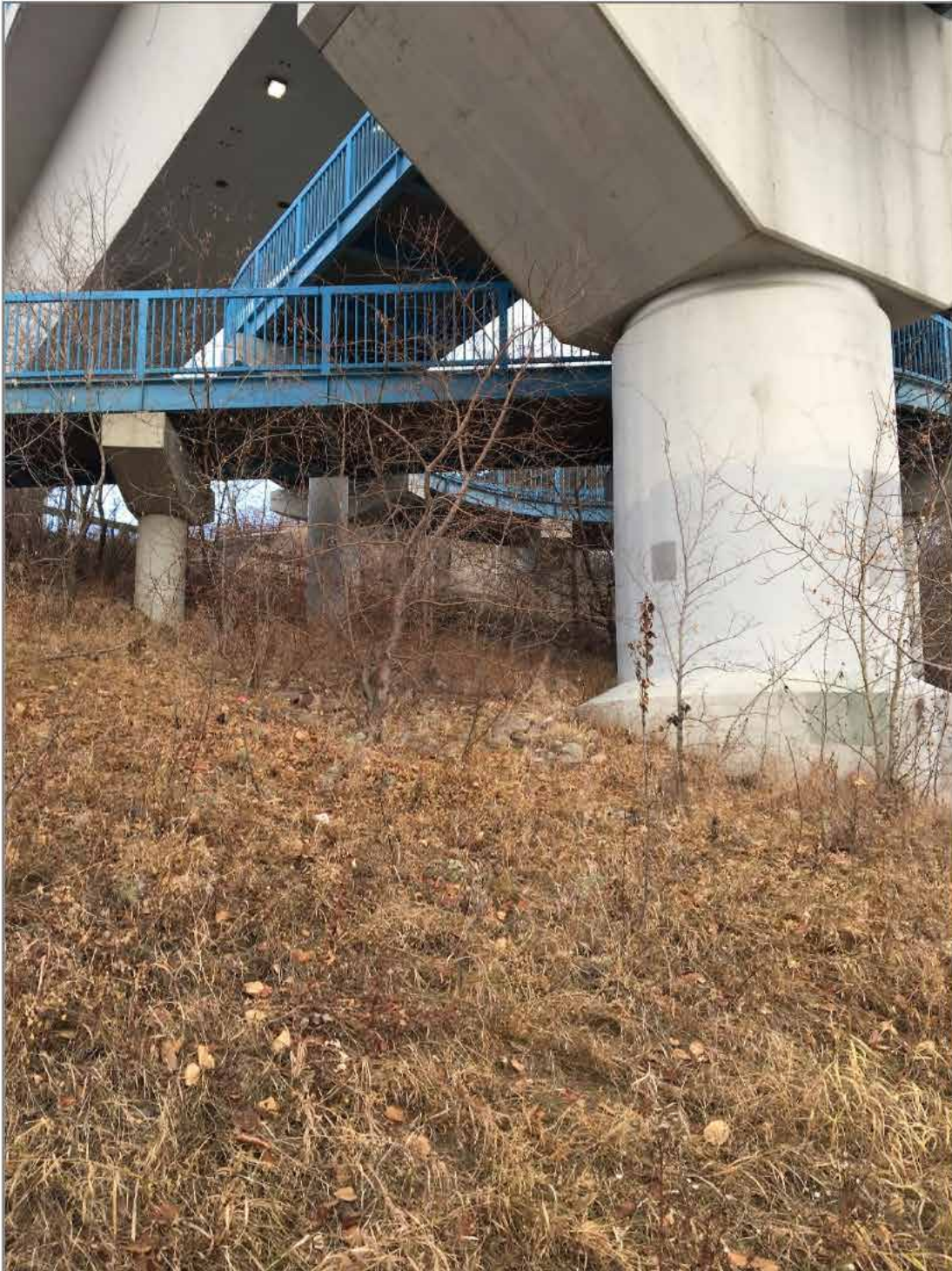
Photo 14: Piers of Existing Footbridge and LRT Bridge
