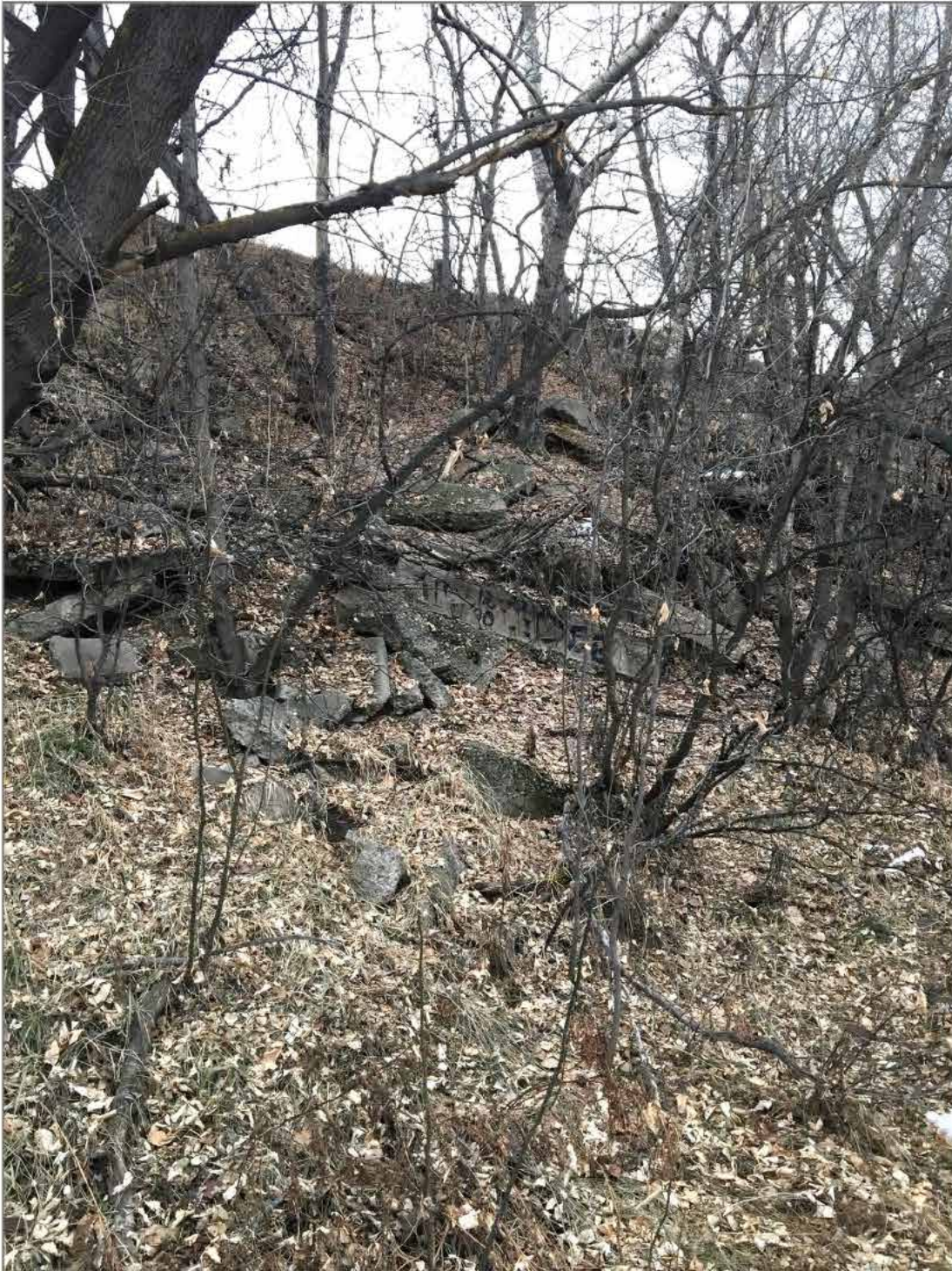
Photo 10: Large Concrete Blocks on River Bank Slope
