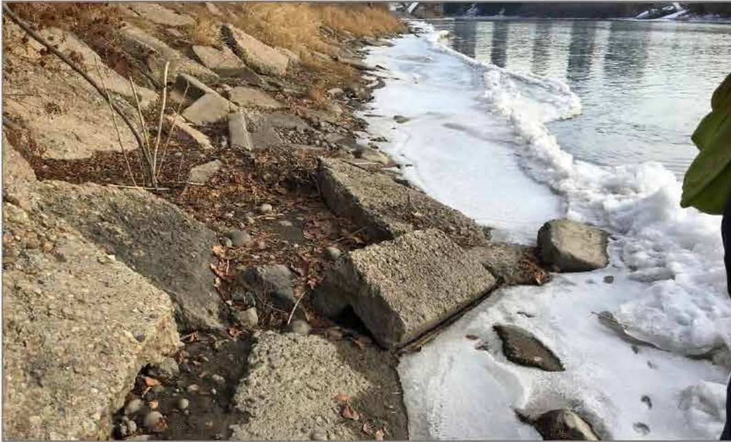
Photo 12: Large Concrete Blocks close to River Level
