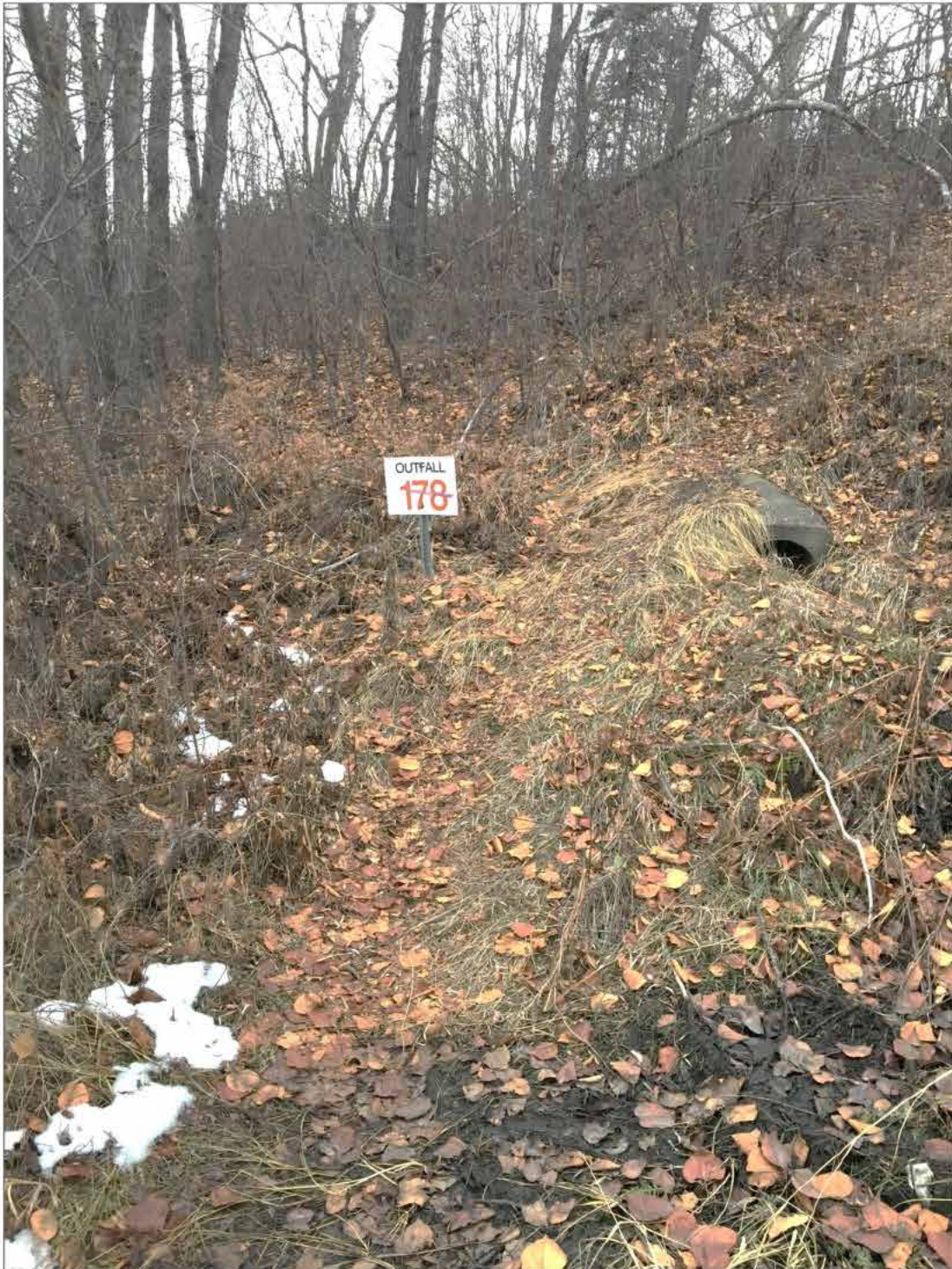
Photo 1: Outfall 178 at Mid-height of River Bank Slope
