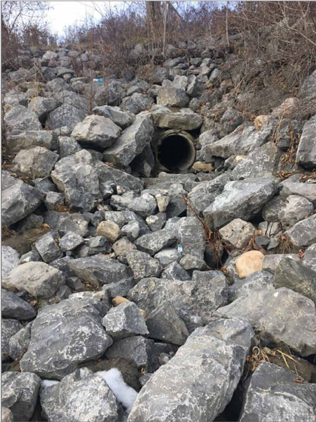
Photo 2: Outfall 33 with Rip Rap Protection
