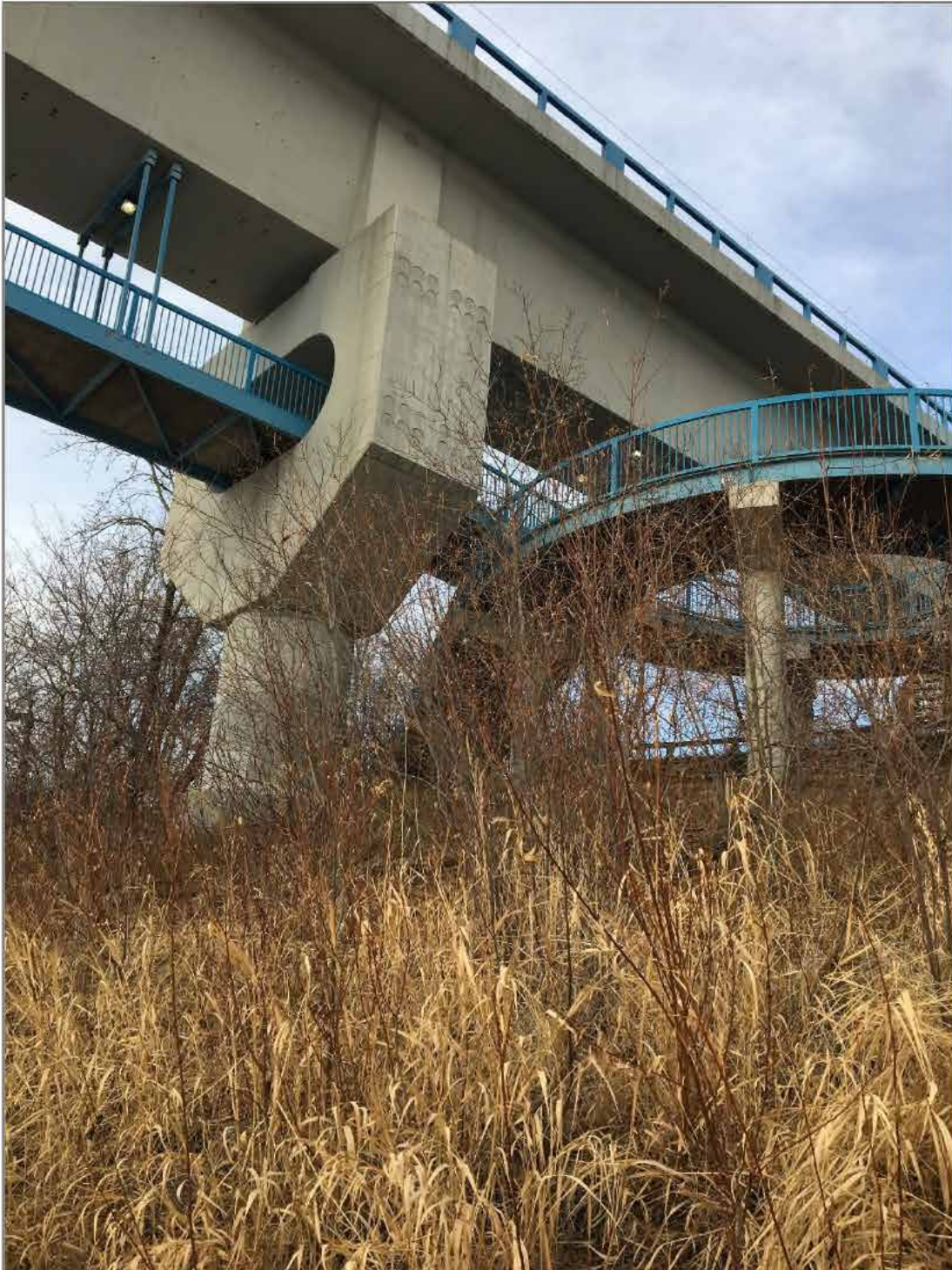
Photo 15: Piers of Existing Footbridge and LRT Bridge
