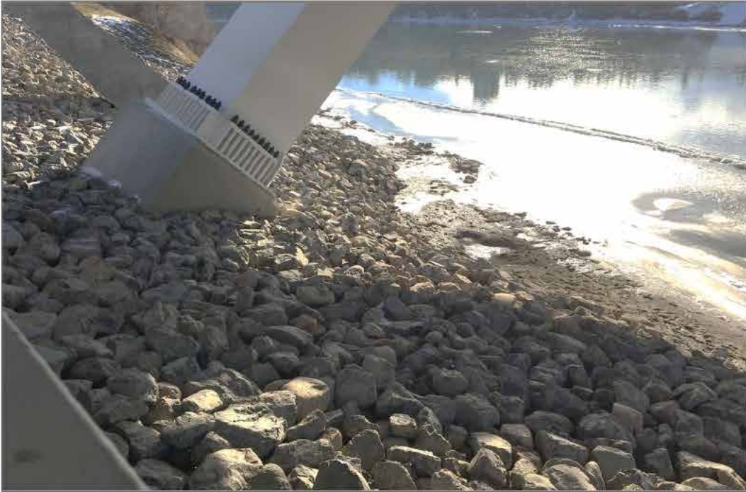
Photo 18: Rip Rap at Walterdale Bridge Abutment
