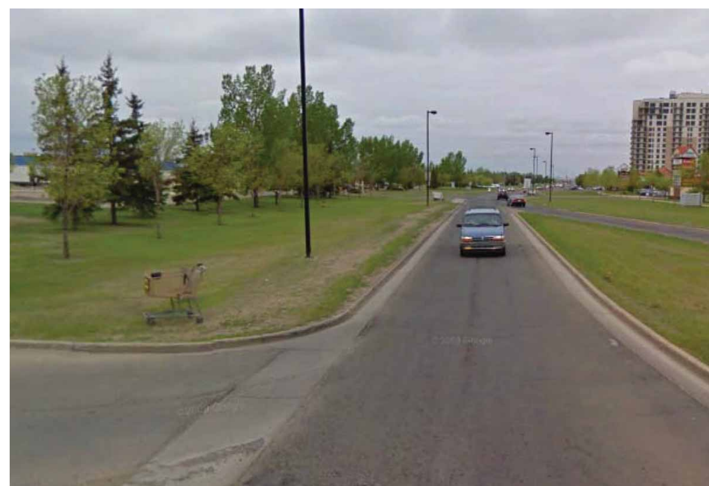
View A - Existing Condition
