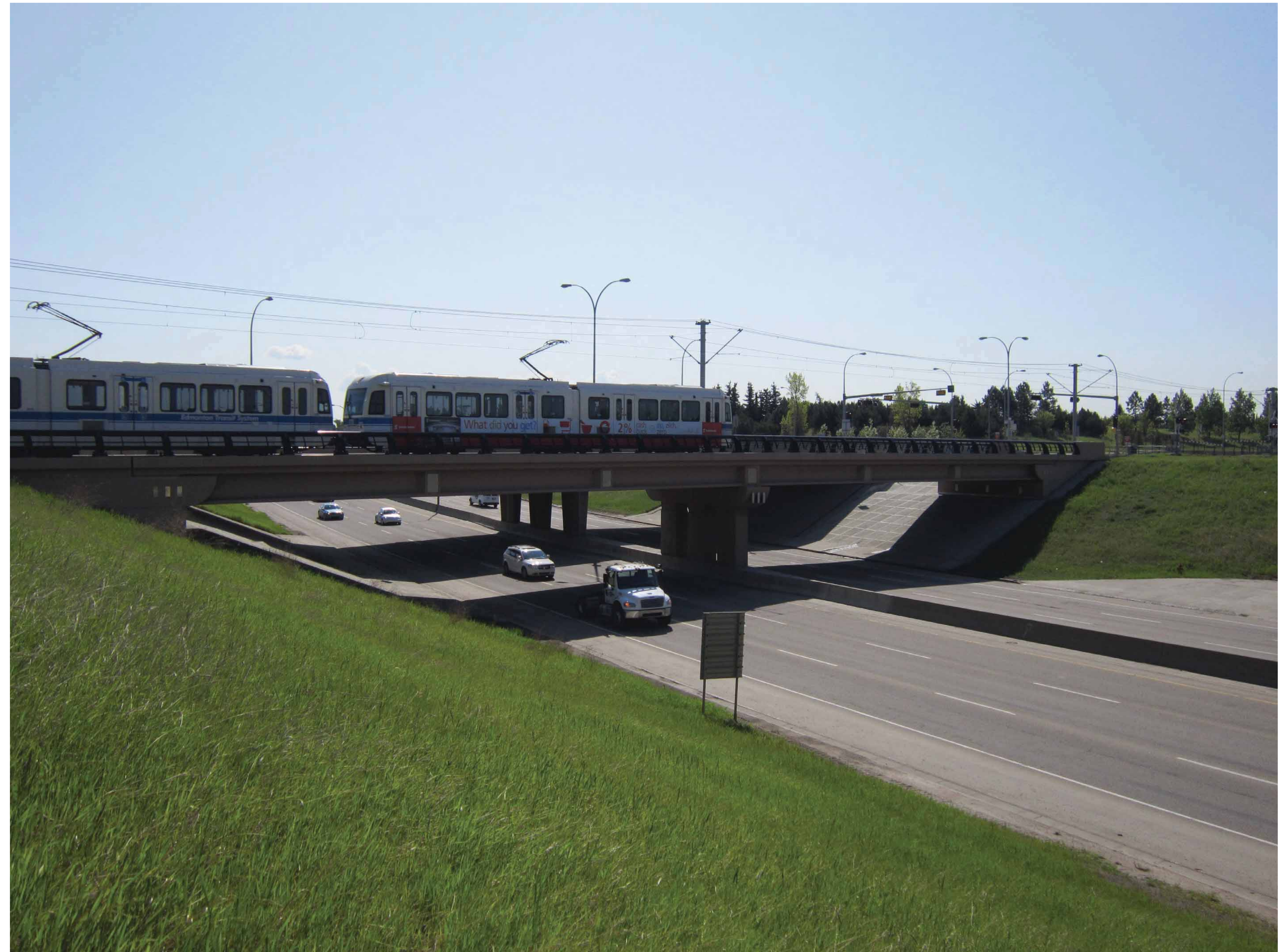
Existing South LRT bridge over Whitemud Drive at 111 Street
