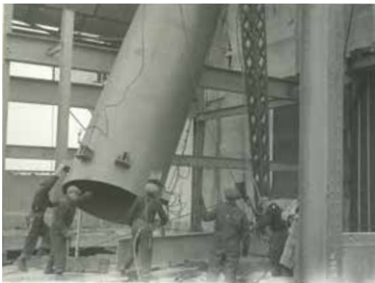
1938 Smokestack install credit Poole Family Archives (EEP)
