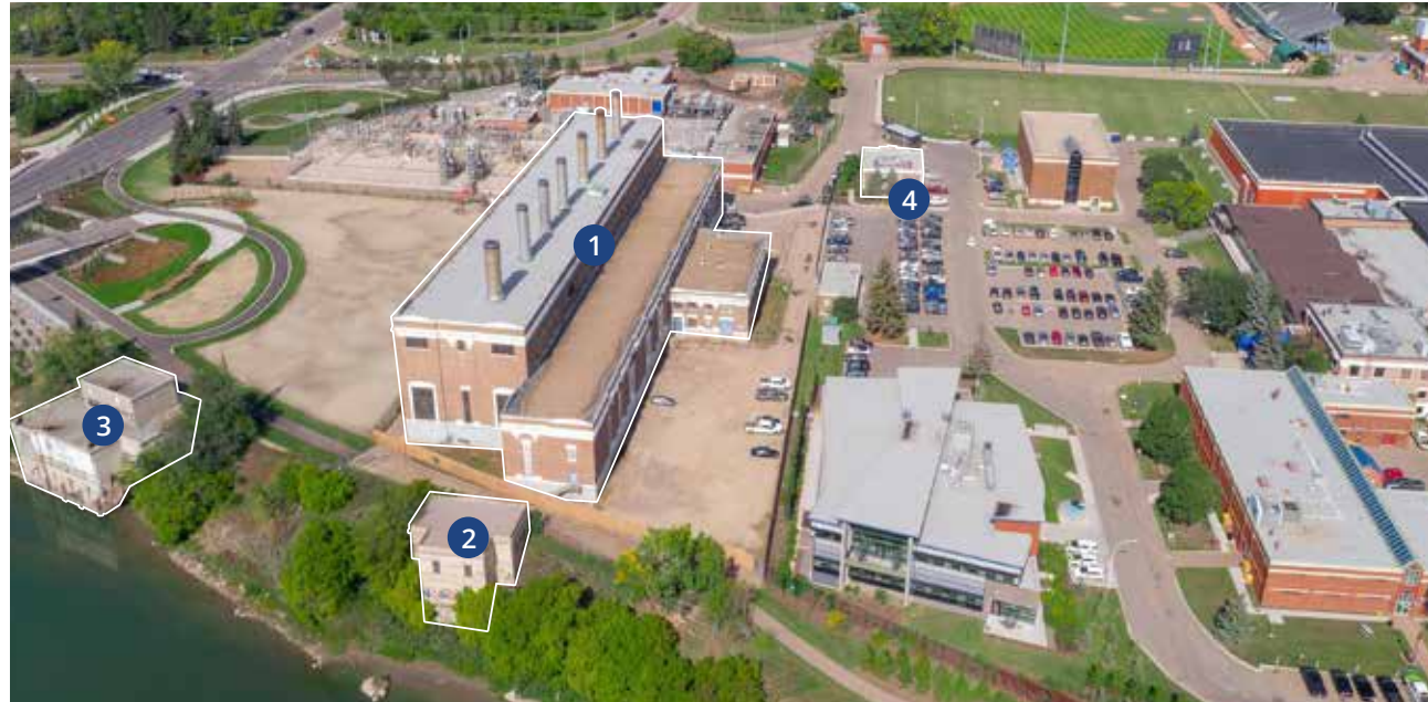
Figure 5 - Rossdale Power Plant
