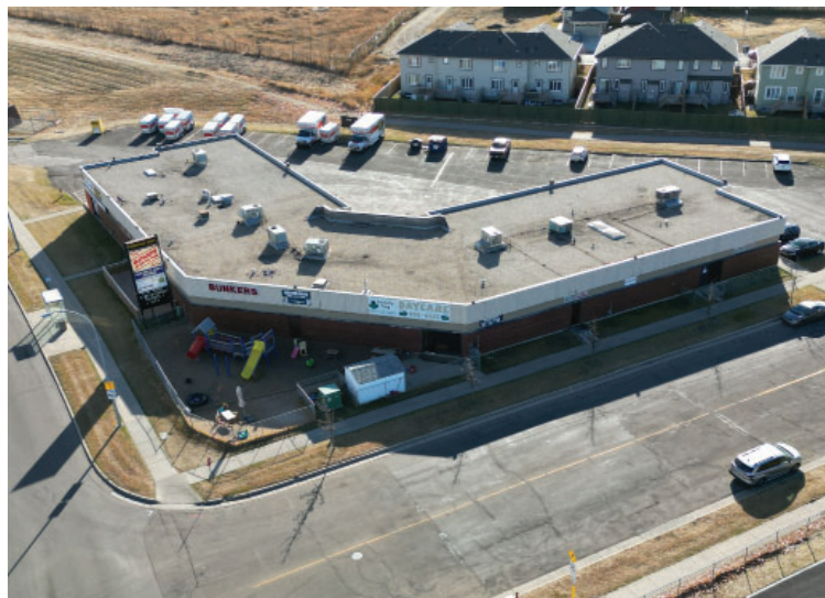
Inward facing commercial site at 127 Avenue and Hermitage Road
