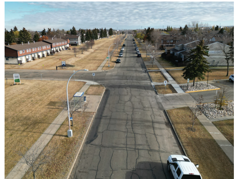
Aerial view of Hooke Road,
