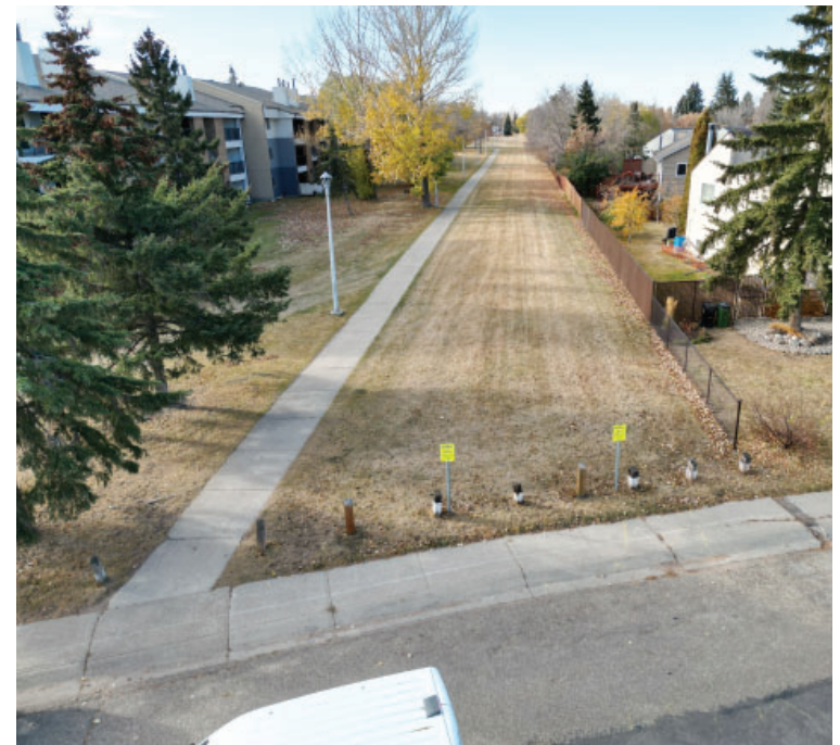
Breezeway with walkway and pipeline corridor
