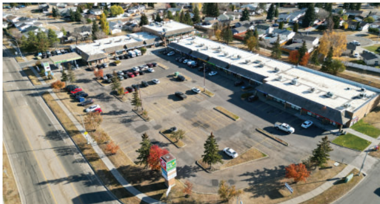
Strip Mall at 40 Street and Hermitage Road
