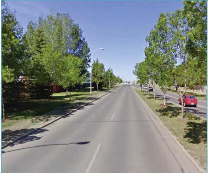
Photo and Cross Section: 153 Ave - 121 St to 127 St (Looking West)
