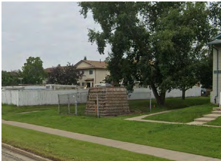
Gas facility near Mill Woods Road
