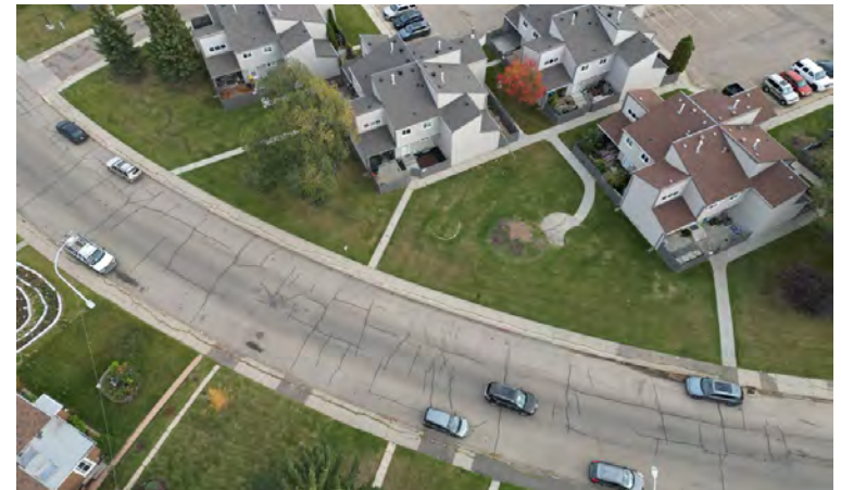
View of Lakewood Road South (11.6 m Wide Collector Road)
