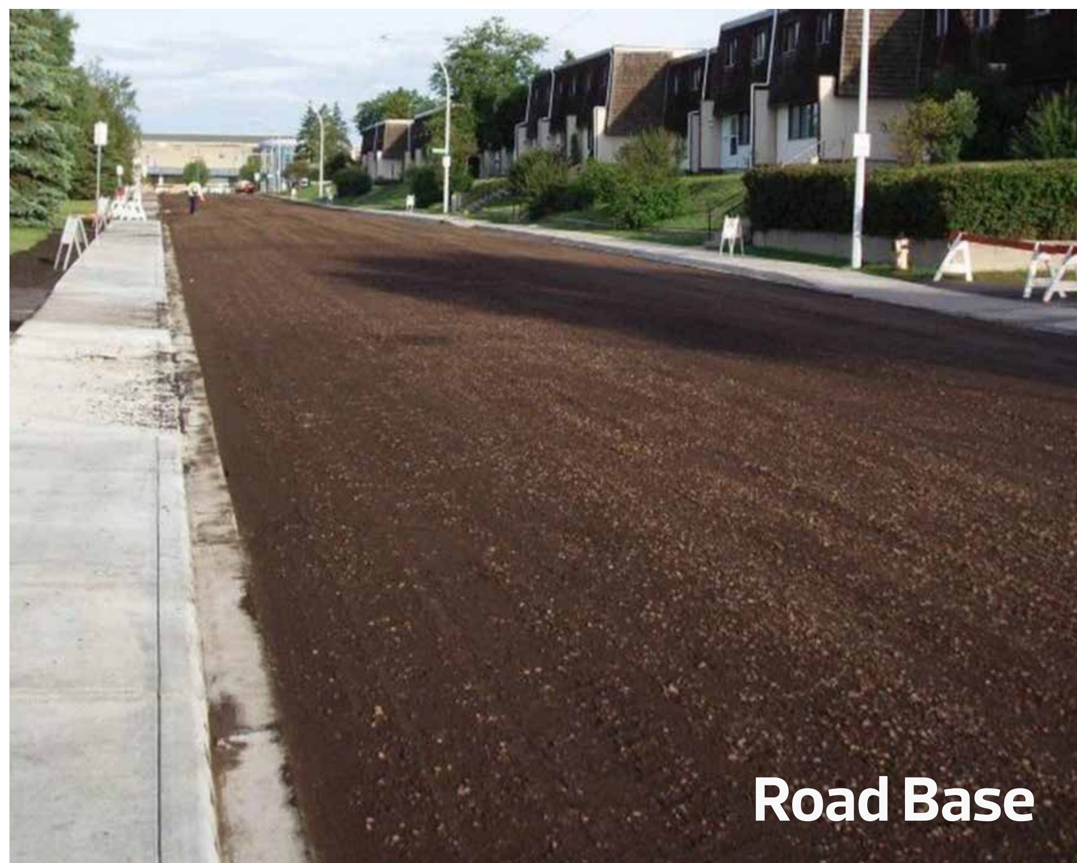
Pulverizing and Mixing the Road
