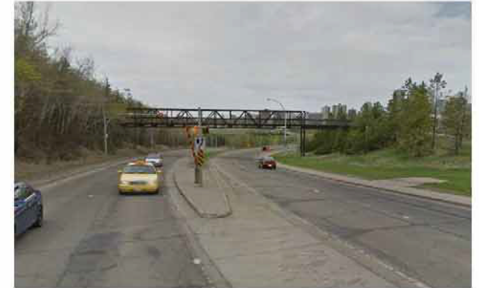
Existing Conditions (Looking west)
