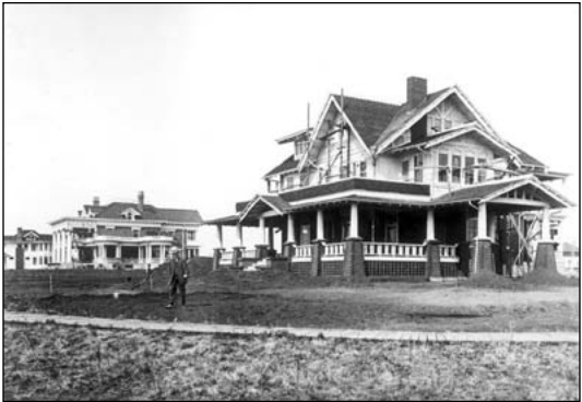
Ada Boulevard houses under construction, 1913. (GAI NA-1328-1136)
