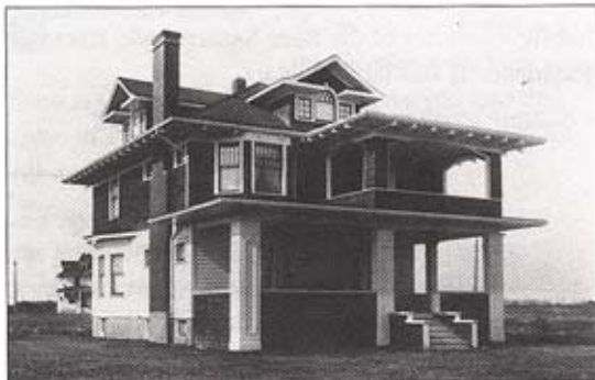
The Field Residence rear, under construction, 1913. (GAI NA-1328-2999)
