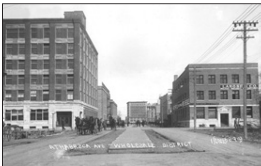
The McKenney Building (right) one year after completion, 1913. (PAA B4944)
