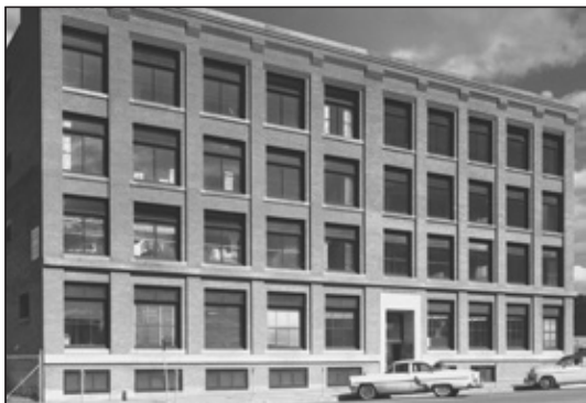
The original Horne and Pitfield Building (right) and its larger annex (left), 1958. (PAA Ws184)
