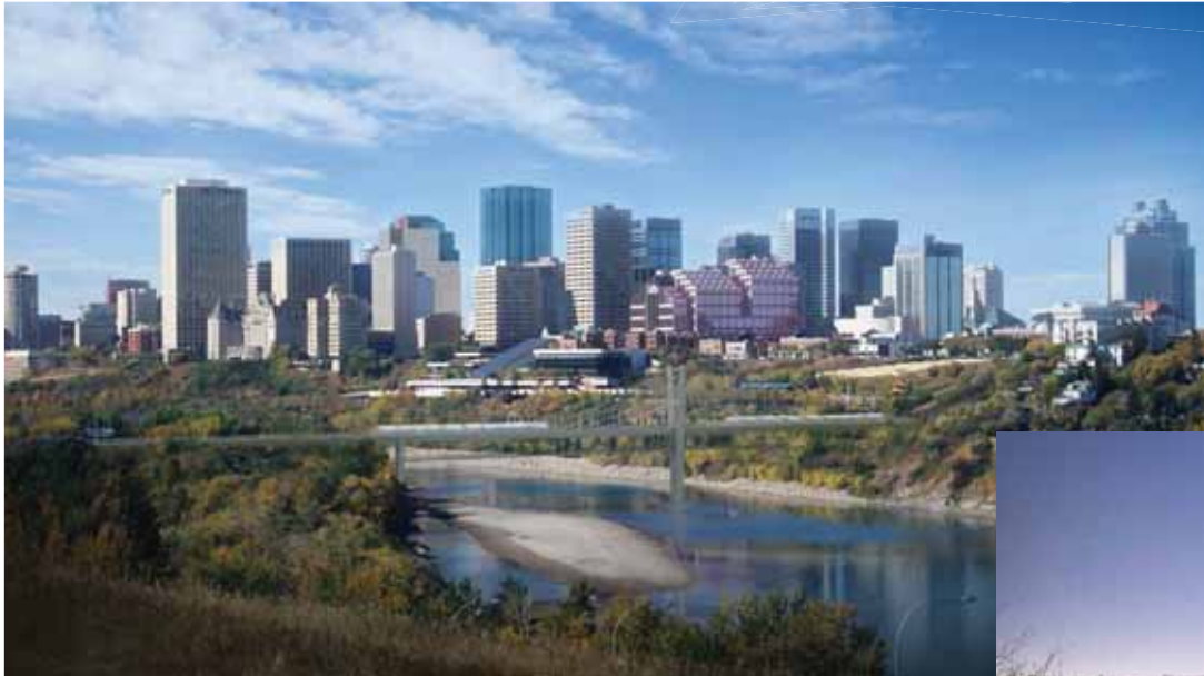
Tawatinâ Bridge looking Northwest
