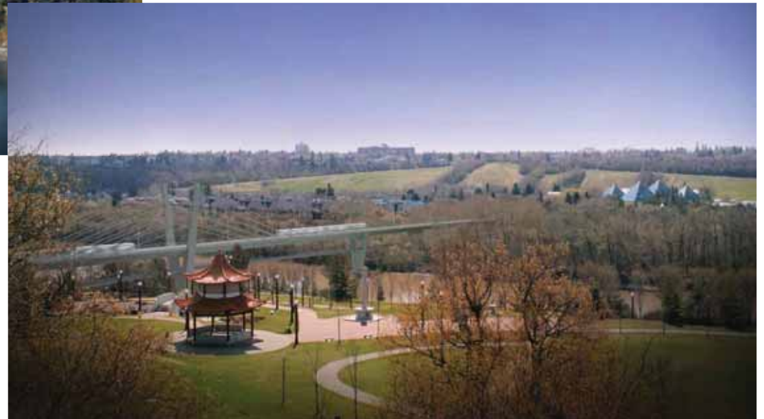
Tawatinâ Bridge looking Southeast
