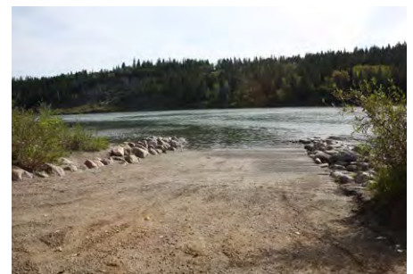
Fig.7: Boat Launch Ramp
