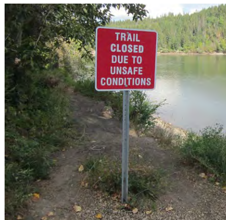
Fig.8: Trail closure due to bank erosion
