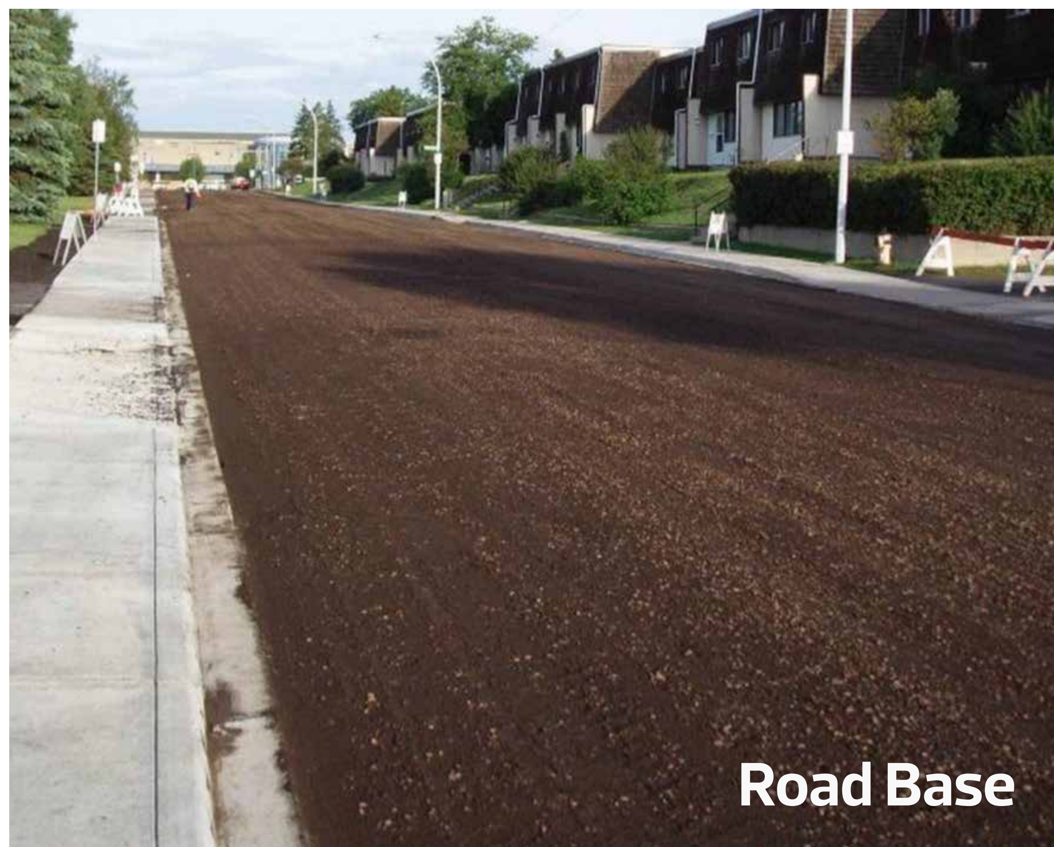
Pulverizing and Mixing the Road
