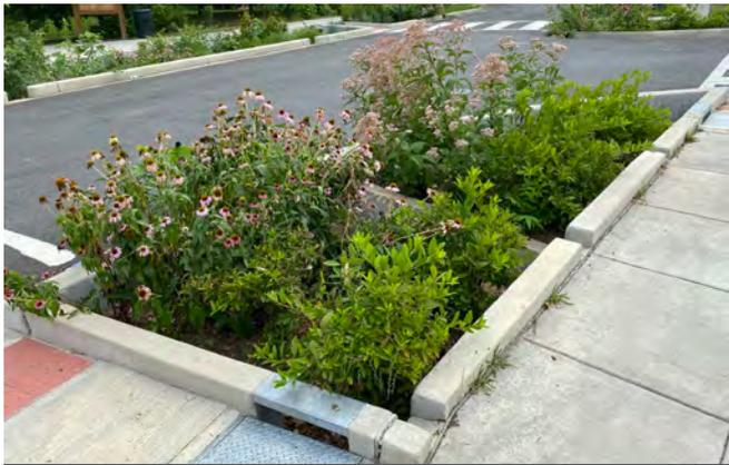
Example of green stormwater infrastructure in a curb bulb
