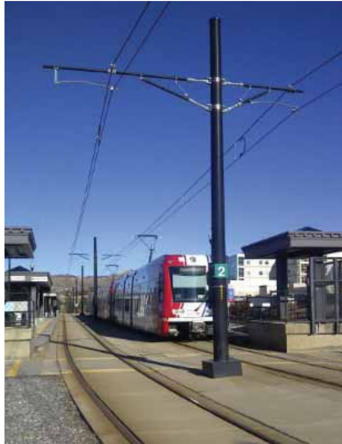
Examples of potential catenary poles
