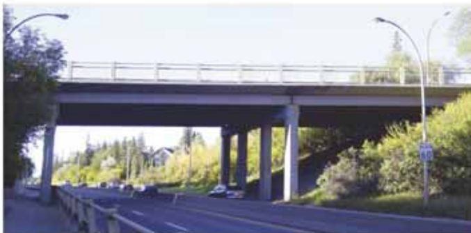
Existing bridge over Groat Road
