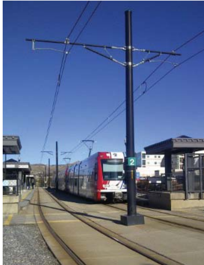
Examples of potential catenary poles
