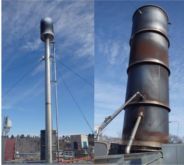
8. The flares are primarily used to control biogas pressures and volumes within the anaerobic digesters headspace.
