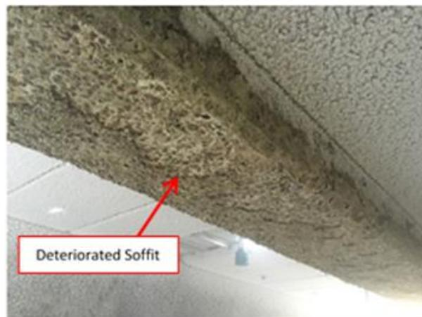
14. The issues were due to extensive hydrogen sulphide ( $H_2S$ ) attacks on the structure.  $H_2S$  is an odorous and corrosive gas, which is emitted from the wastewater stream due to
