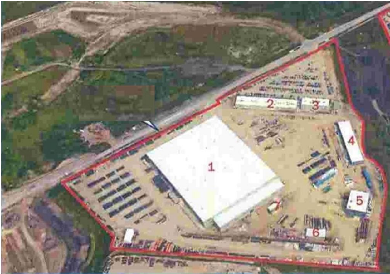
Figure 3.0-1 Aerial View of the Aurum Property
