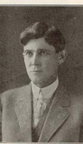
J. C. Hoffman, Supt. of Power Plant EB-26-429
