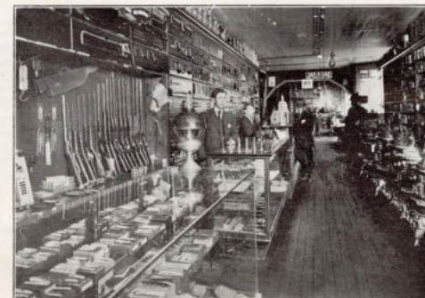
INTERIOR OF JASPER AND THIRD ST. STORE
