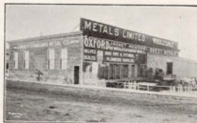
OFFICE AND WAREHOUSE, ATHABASCA AVE.
