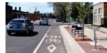
Unprotected one-way bike lane on road
