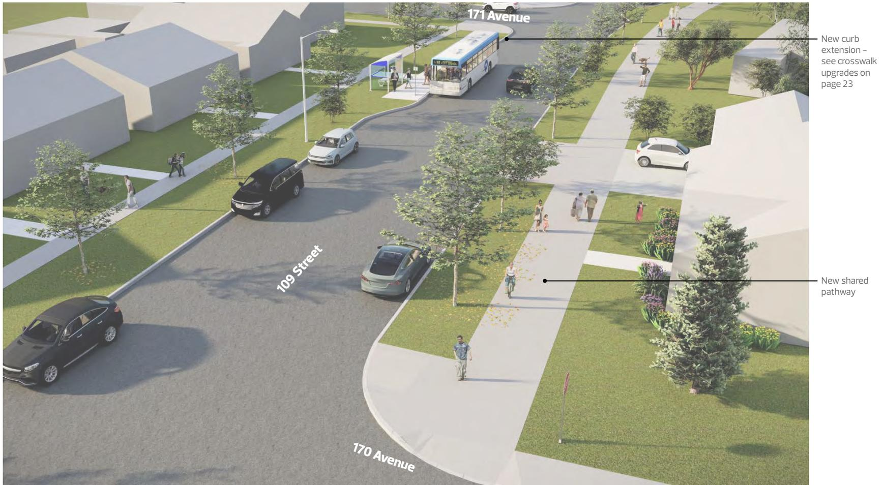
Figure 21. New shared pathway along the internal loop road (109 Street between 170 and 171 Avenues)
