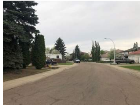
1 Local Residential Road
