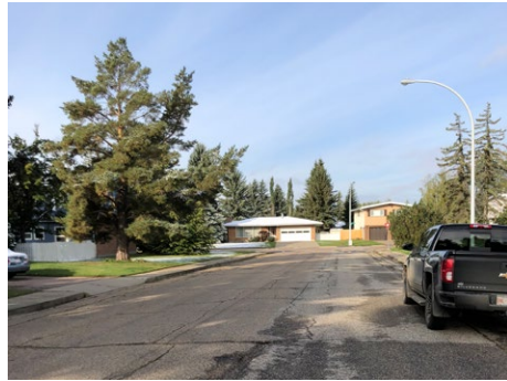
1 Local Residential Road
