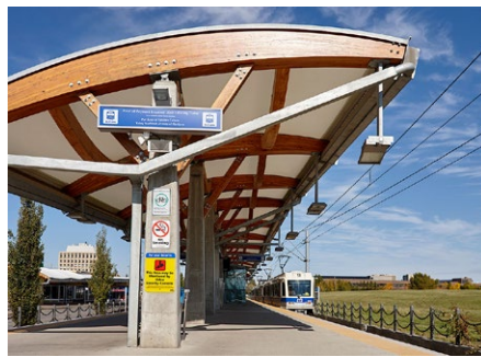
2 South Campus/Fort Edmonton Park LRT Station
