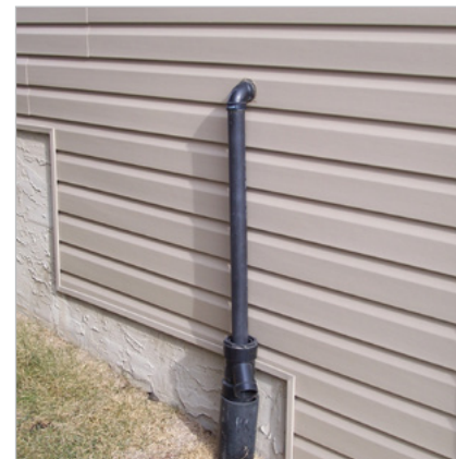
Sump Pump to storm service multi-family site
