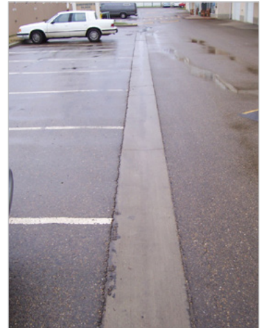
Concrete swale in a parking lot
