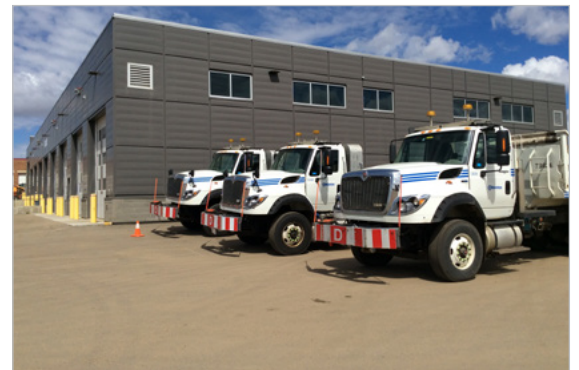
Lot grading with slope away from a building on hard surface.
