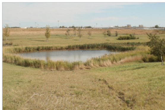
Stormwater Facility at a Commercial/Industrial Area
