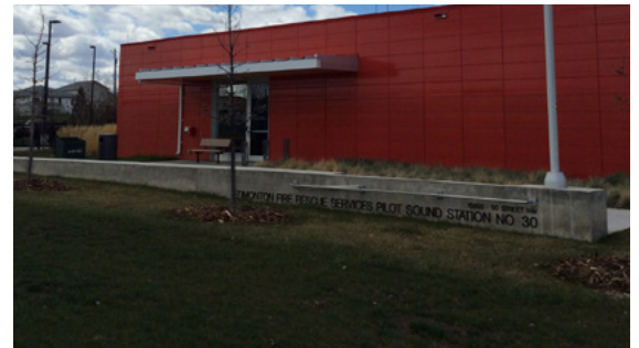
Lot grading with slope away from a building on soft landscaping.
