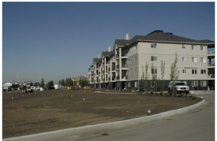
Final Grading in progress at a condominium / multi-family site
