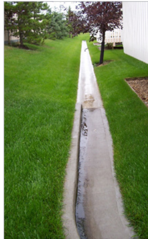
Concrete drainage swale
