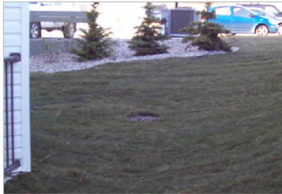
Grass swale and catch basin at an apartment site
