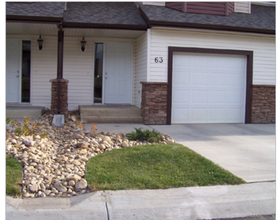
Grading away from the wall on a row housing project
