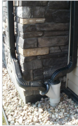
Downspouts at an apartment connected to storm service
