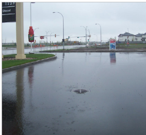
Drainage into a catch basin during a storm
