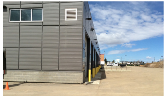
Grading away from a Commercial Building on hard surface
