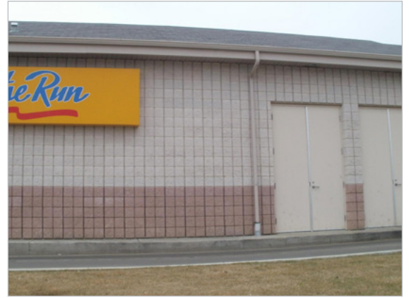
Downspout at a commercial property connected to storm service
