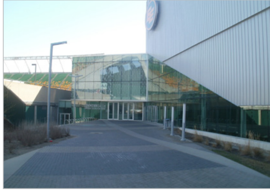
Grading of hard surface (paving stones) with slope towards a catch basin
