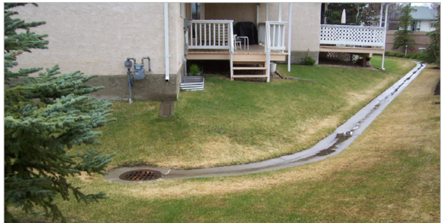
Condominium site concrete drainage swale that drains into a catch basin
