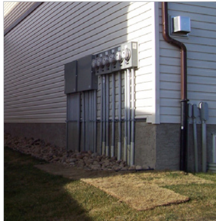
Positive slope away from building
