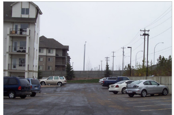
Example of asphalt grading on a condominium parking lot
