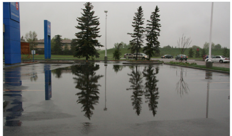
Ponding area around a catch basin on private property during a storm event
