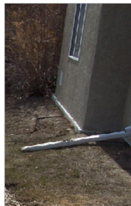
Downspout and extension at an apartment
