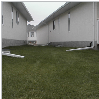
Downspouts with extensions at condominium
