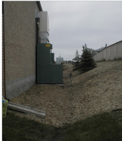
Internal drainage swale
