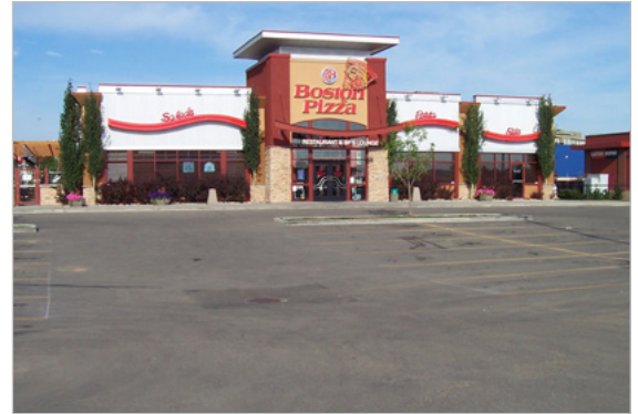
Asphalt repair around the catch basin
