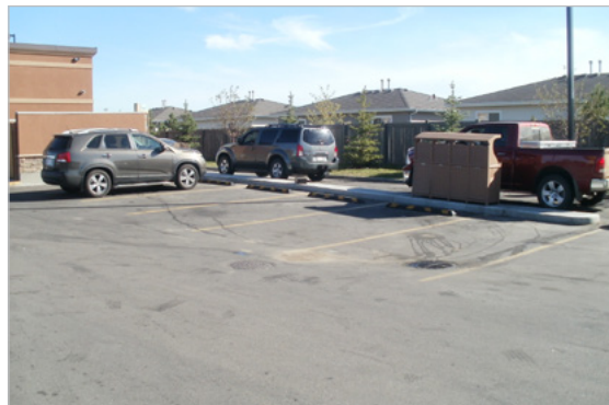
Surface drainage is controlled to drain towards private catch basins
