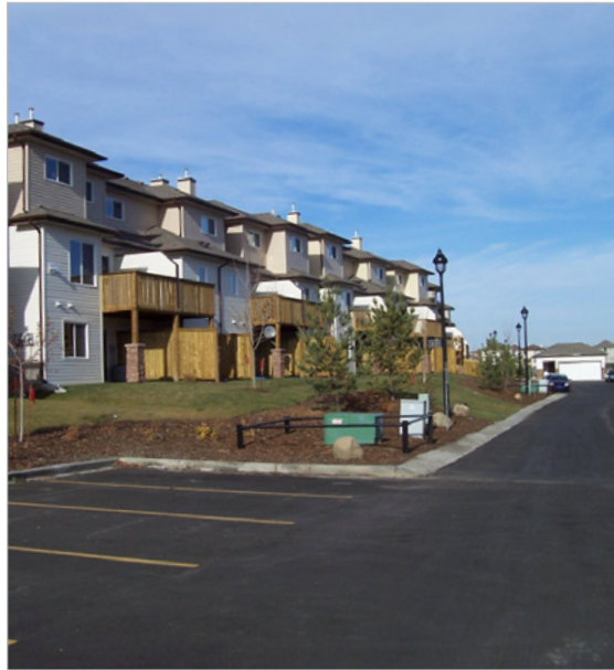
Lot Grading slopes away from a Multi-Family buildings
