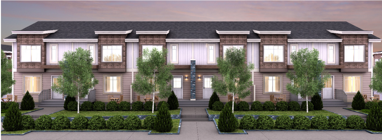
Laurel 2.5 Storey (under construction) and alternate colour scheme 2215 24 St. NW
