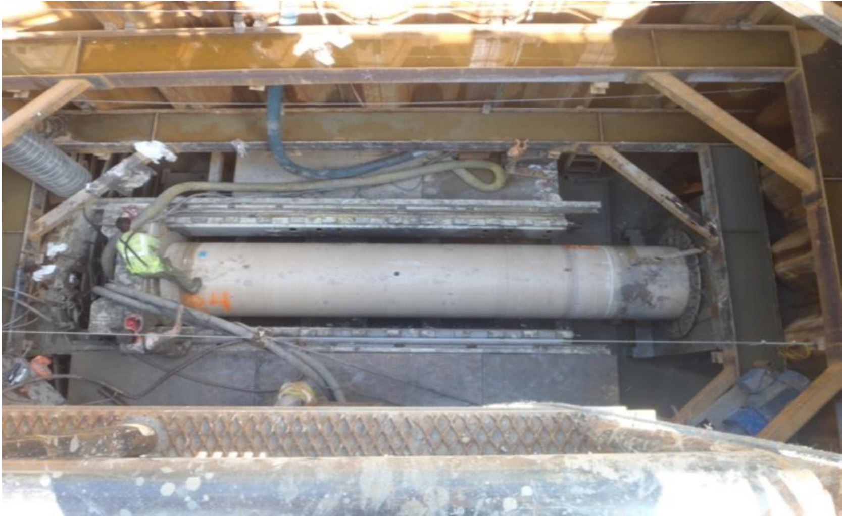
Figure 4. WESS W14 – Micro Tunneling Construction
