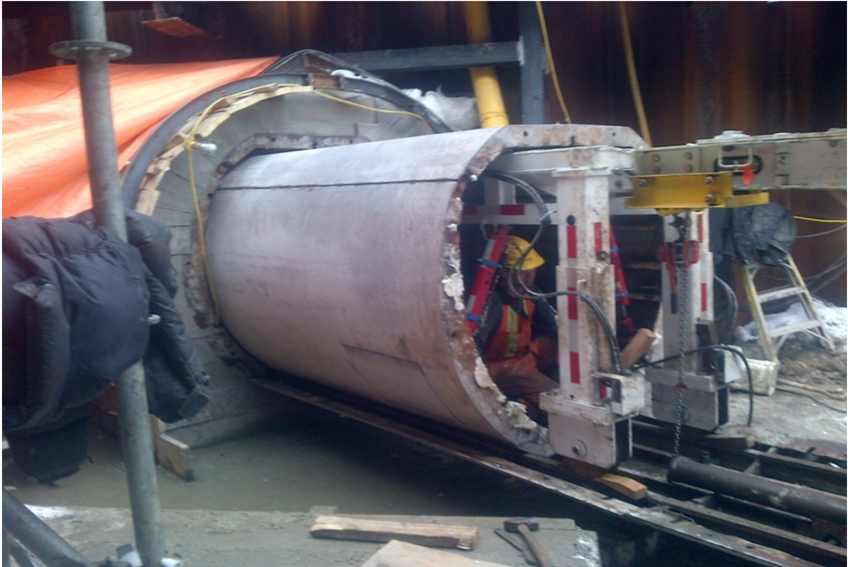
Figure 1. SESS SA1 – Construction Area
