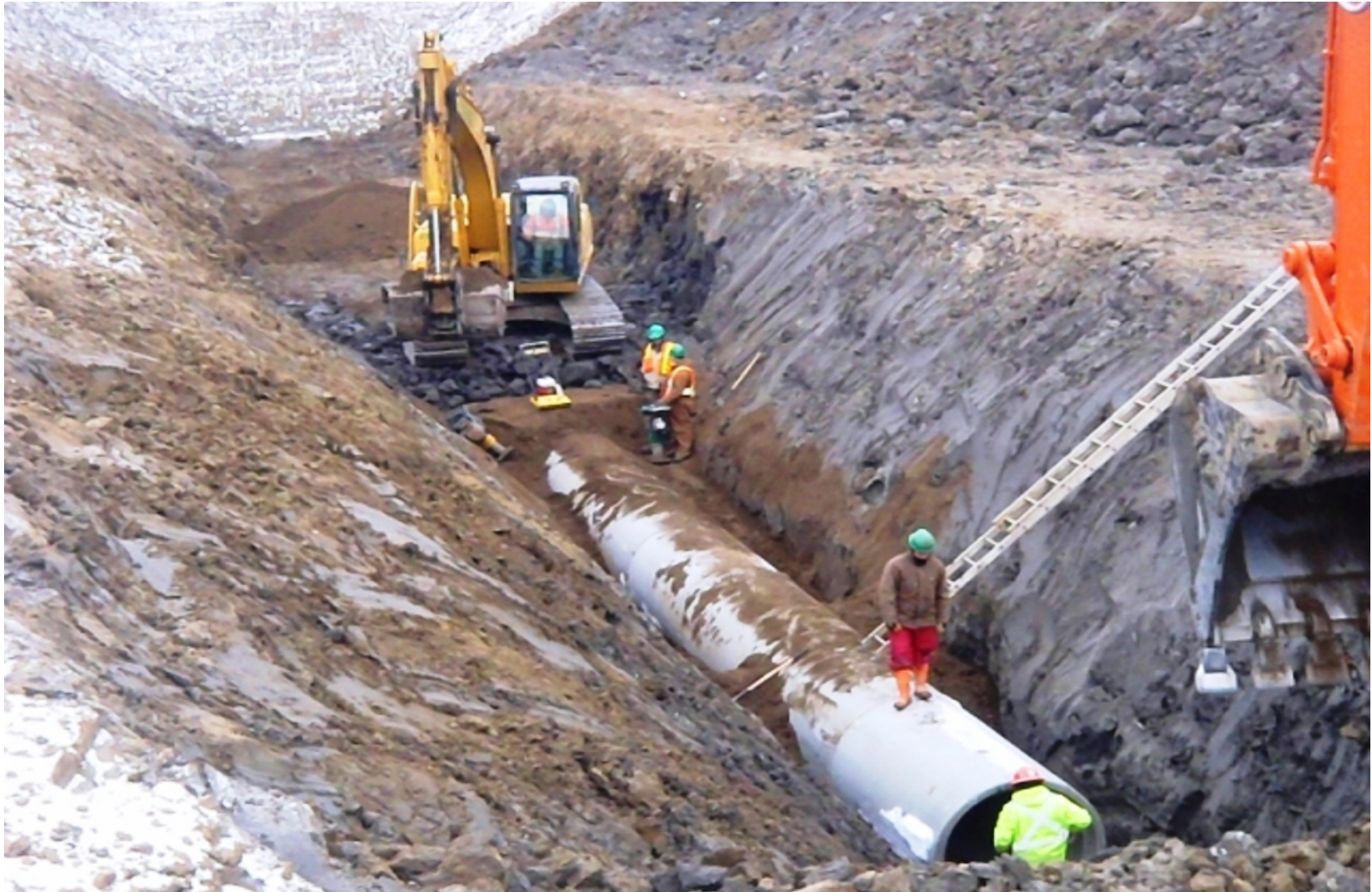
Figure 2. SESS SE4a – Backfilling of the SE4a sanitary trunk.
