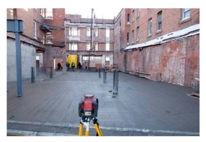
This picture shows the interior of the Lodge Hotel after demolition of the interior wooden structure. The basement foundation has been poured and the roof removed.
